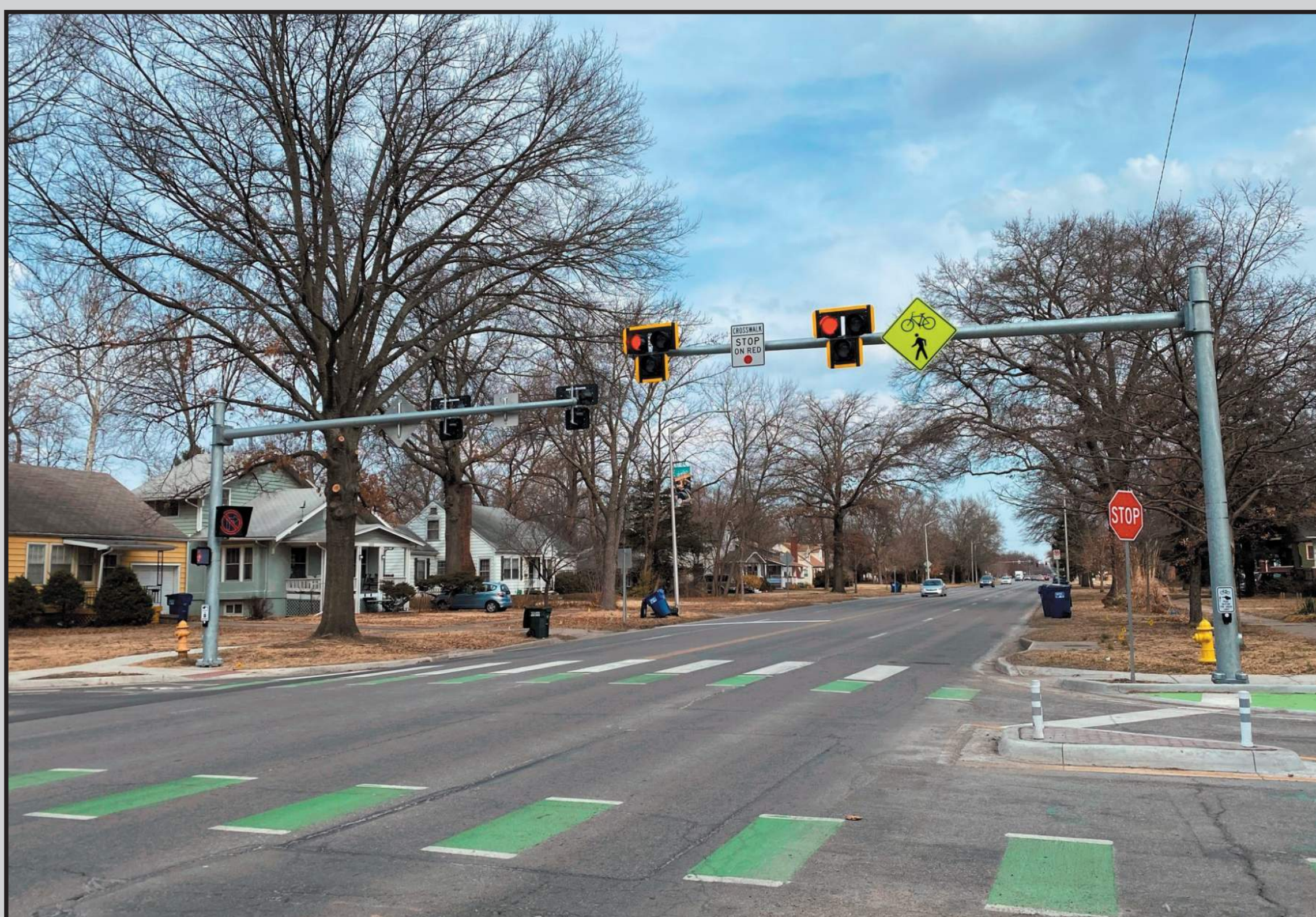
Example of how a HAWK signal may function at the intersection of 17th & Mass Example location: 21st & Mass Street | HAWK signal
