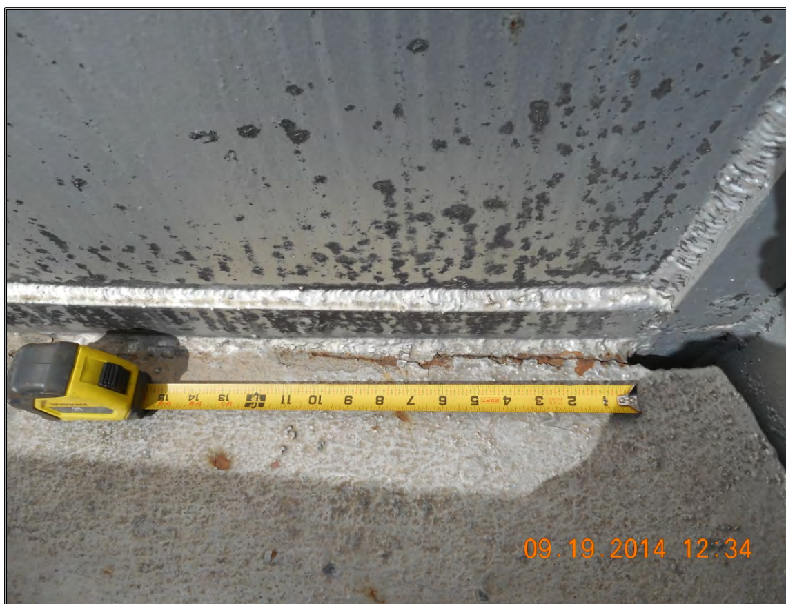
Photo 21: Crack in Balcony Checker Plate.
