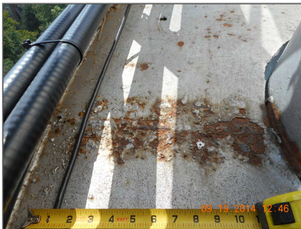
Photo 23: Deep Pitting of Checker Plate Over Support Bracket.
