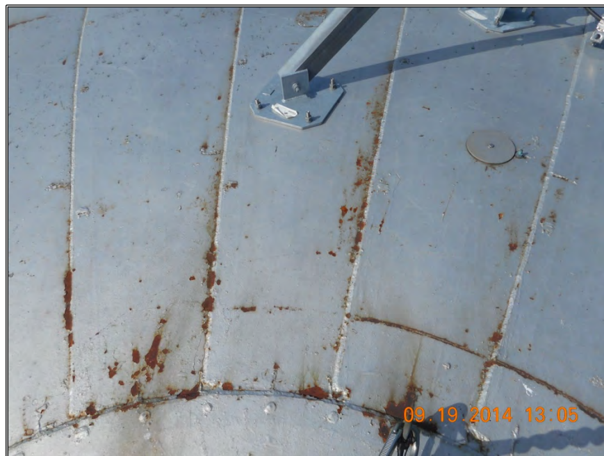
Photo 15: Exterior of Lap Welded Top Shell.
