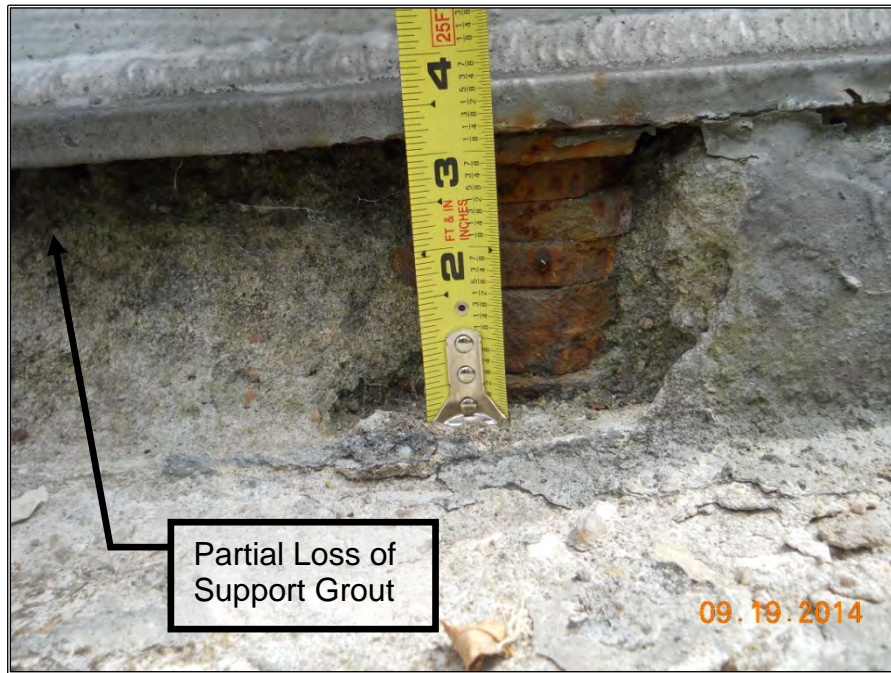
Photo 6: Close Up View of Grout Loss. Original Steel Construction Shims are Exposed.
