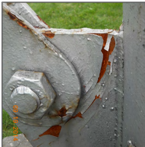
Photo 9: Cracking and Chipping of Coating on Gussets.
