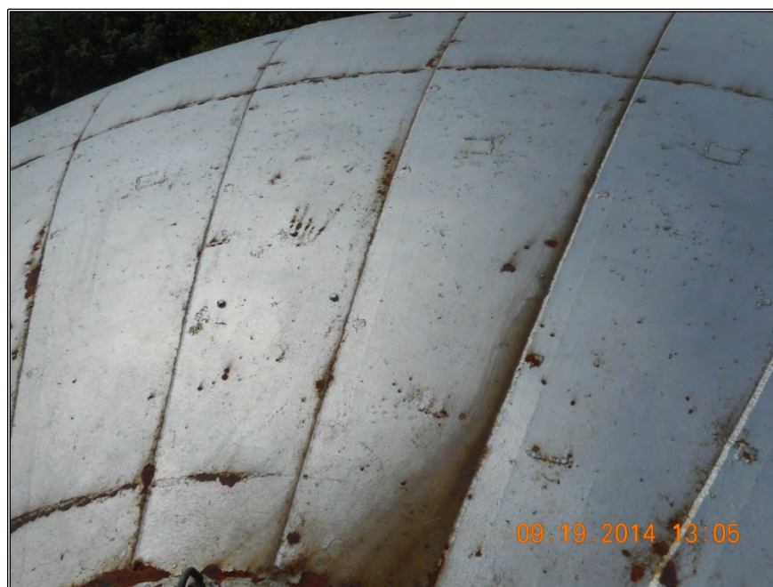
Photo 16: Exterior of Lap Welded Top Shell.
