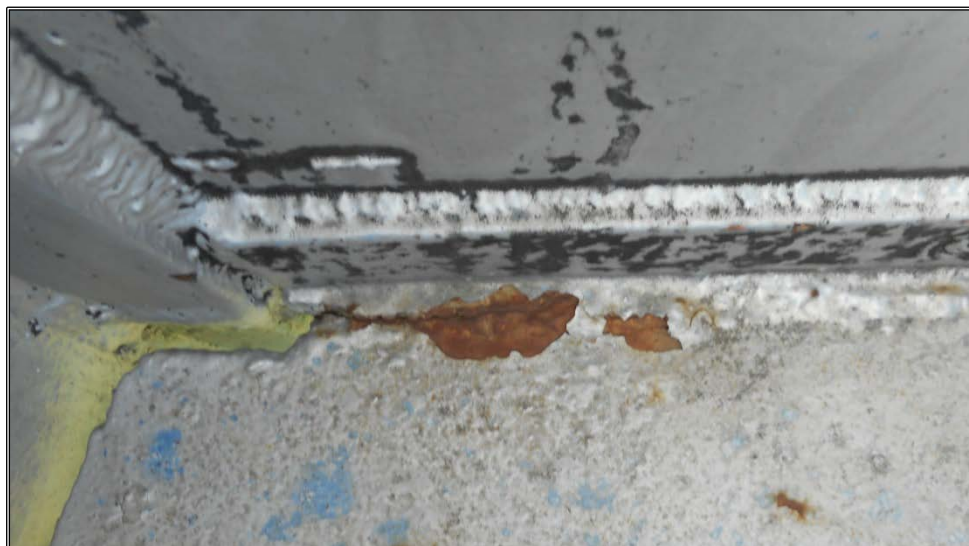
Photo 22: Smaller Crack in Balcony Checker Plate.
