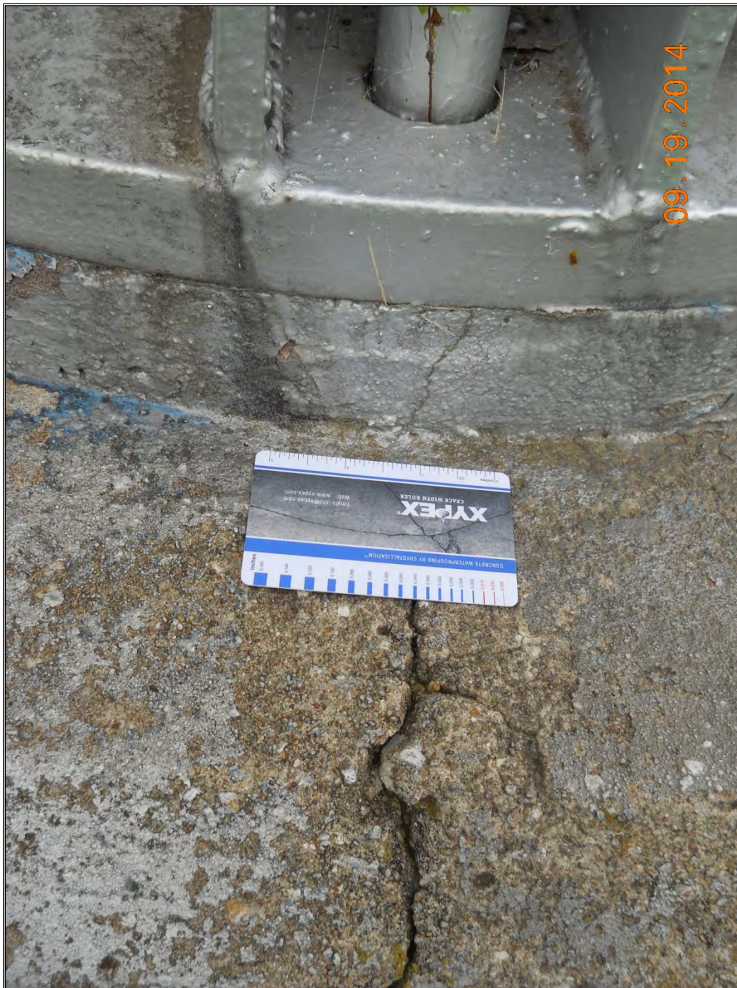
Photo 3: Close up View of 0.05inch wide Crack with Spalling in Footing.
