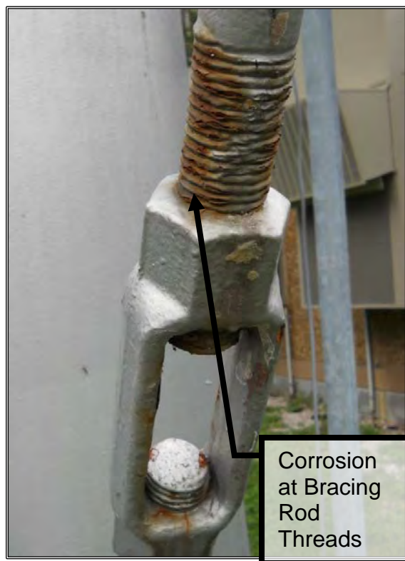
Photo 8: Surface Corrosion on Threaded Bracing Rods.
