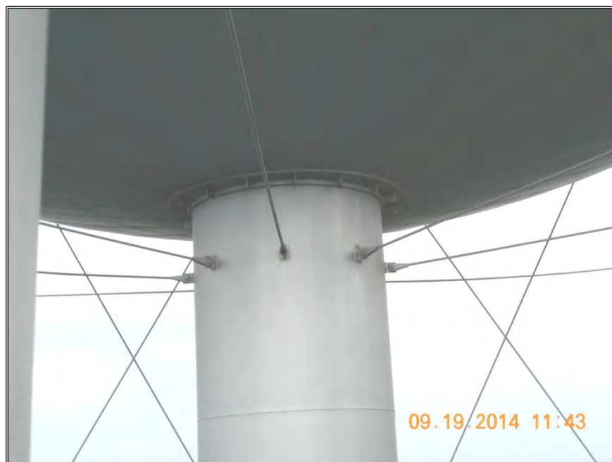
Photo 13: Butt Welded Bottom Shell at Connection to Riser.
