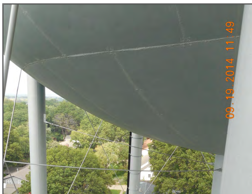
Photo 14: Butt Welded Bottom Shell.
