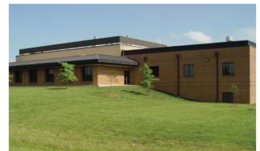
BTBC Expansion Facility
