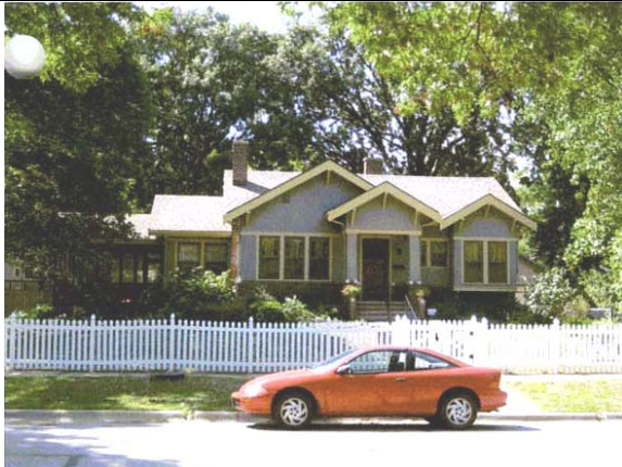
East (front) elevation of 621 Tennessee Street.
