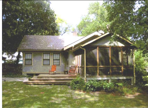
South elevation of 621 Tennessee Street.
