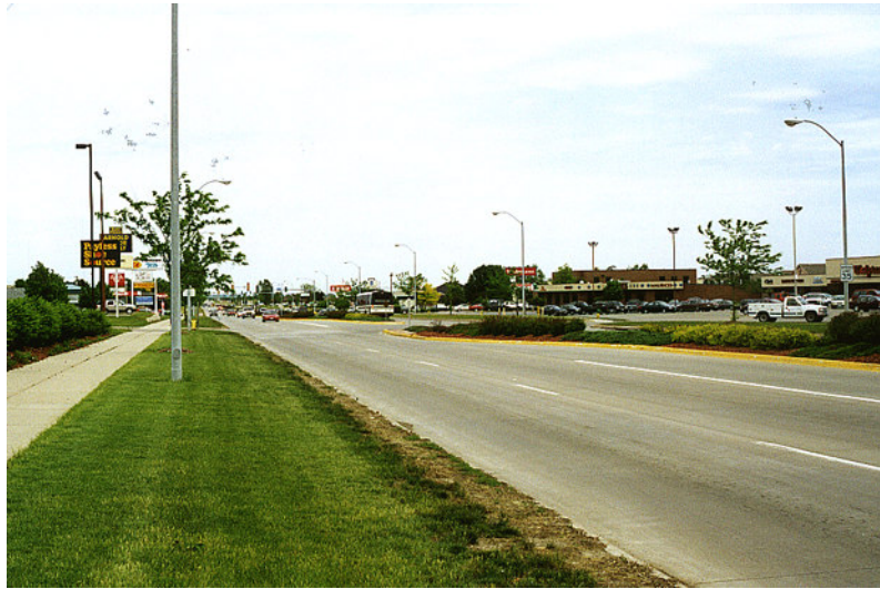
Photo 12 Center median along Highway 69, Ankeny, Iowa
