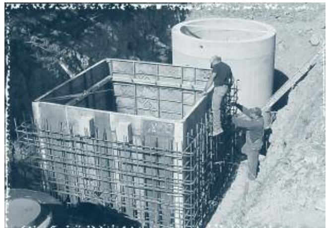
Crews worked on the construction of a southeast pump station.
