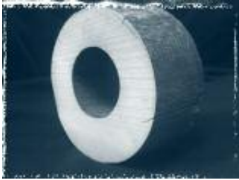
A wooden water main that is said to have been installed between 1865 and 1870.
