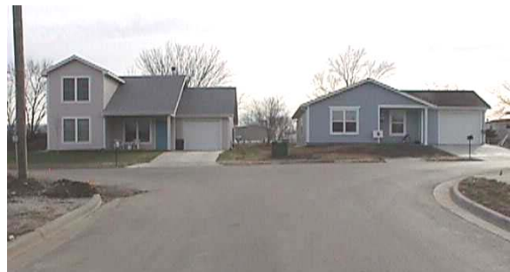
Atherton Court homes built by Tenants to Homeowners and Habitat for Humanity through funds provided by CDBG and HOME programs.
