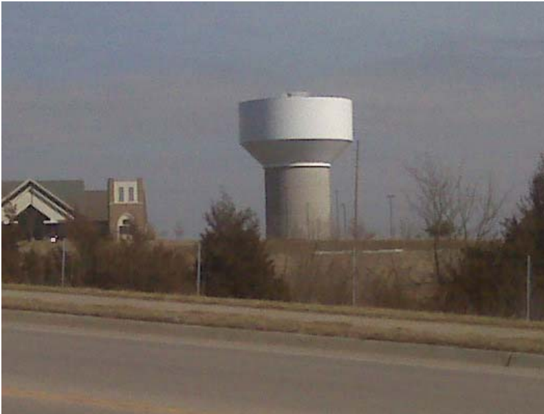
Left: The department raised the bowl on Stoneridge Water Tank in late fall. Stoneridge Water Tank will store 1.5 million gallons of drinking water when done. It is located at the northwest corner of 6 th Street and Stoneridge Drive.
