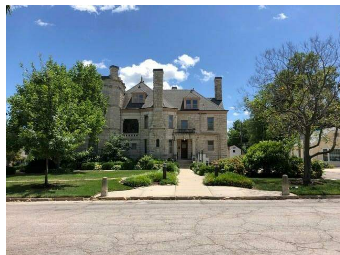
1307 Massachusetts - North Elevation
