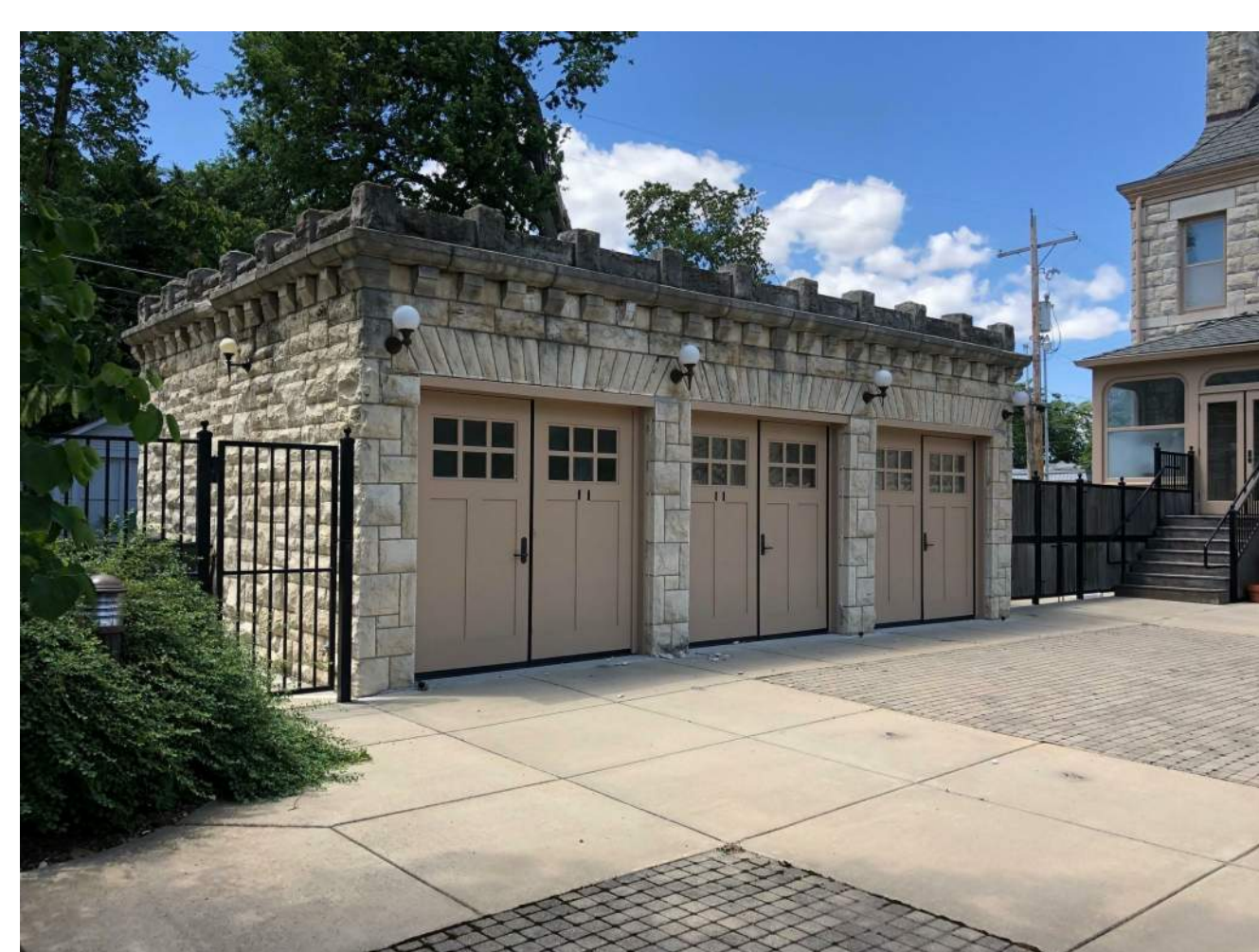
Carriage House - East Elevation
