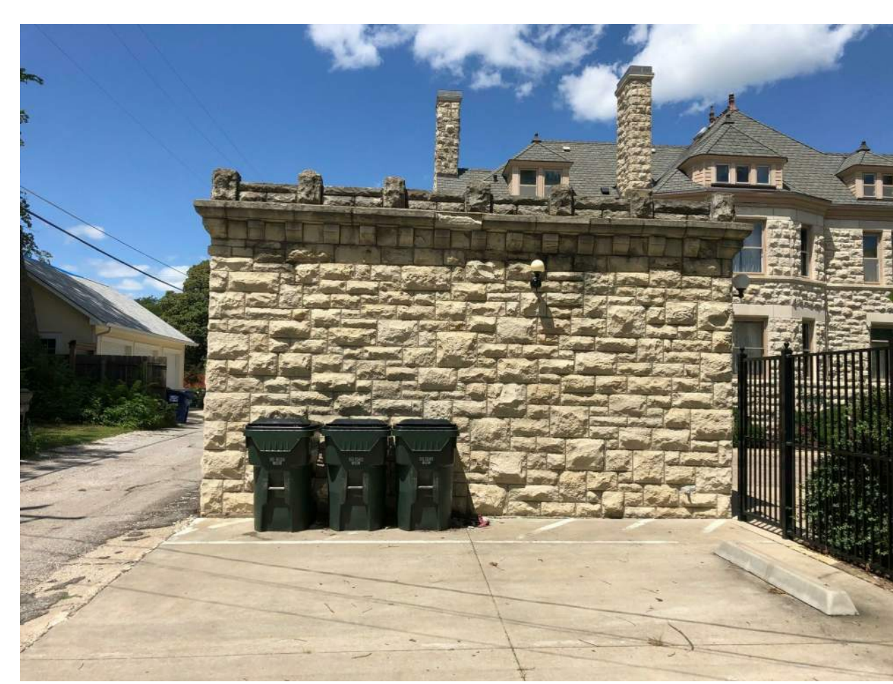
Carriage House - South Elevation
