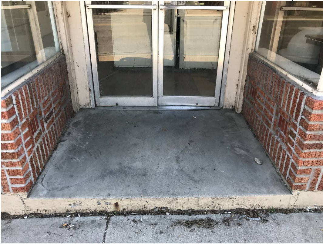
Photo 14: North Façade Looking at Recessed Storefront Entrance
