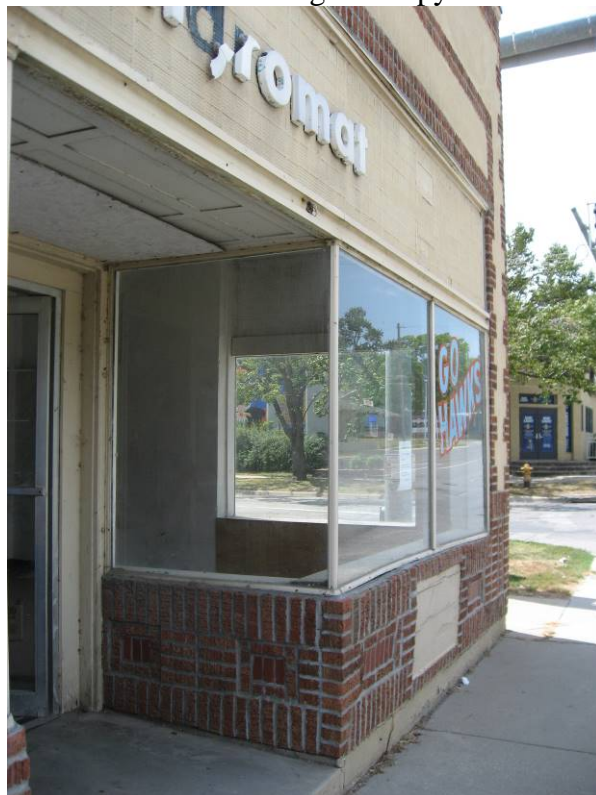
Photo 7: North Façade Recessed Entry Looking West-Southwest
