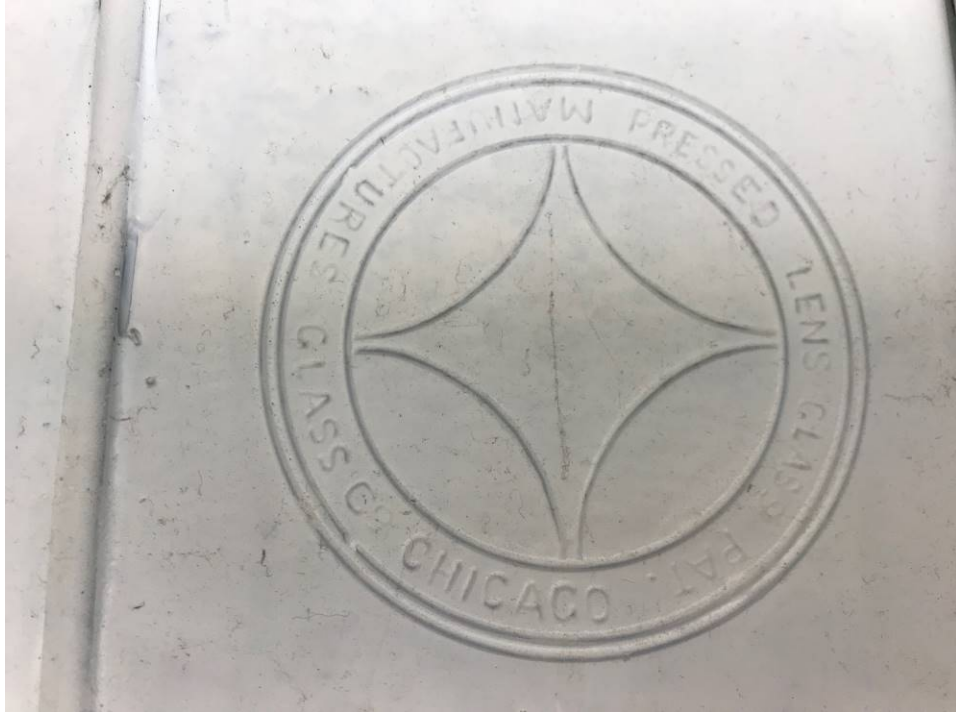
Photo 16: North Façade Detail of Transom Pressed Glass
