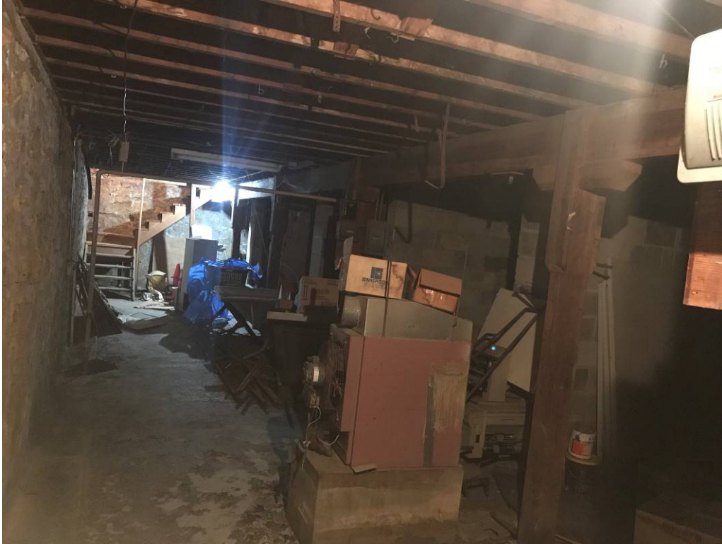
Photo 12: Basement East Area Looking South
