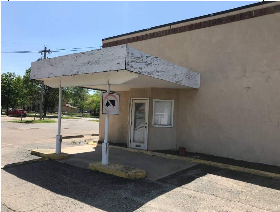
Photo 6: Drive-Through Canopy East Side
