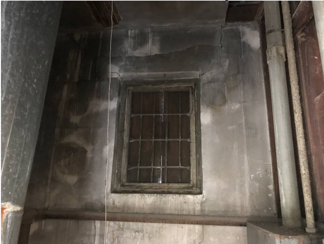
Photo 13: First Story at Southwest Corner Looking West
