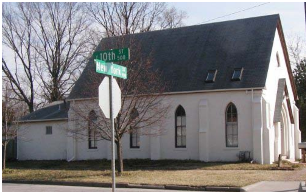
The German Methodist Episcopal Church at 1001 New York Street
