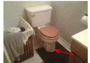
19. Basement Bathroom Ventilation: No ventilation - No ventilation. Recommend consideration be given to installation of a vent.
