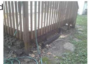
5.  Grading: Minor slope, Negative slope - Grading has settled in areas around the home, allows moisture to accumulate near structure. Recommend repair by a qualified landscape contractor.
