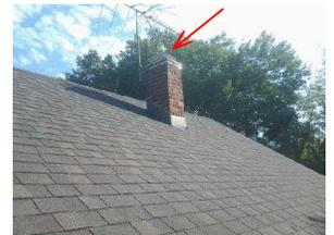
13.      Flue/Flue Cap: Mortar - :Chimney flue cap is not installed. Recommend installation of rain/snow cap to keep moisture and wildlife from entering chimney flue.
