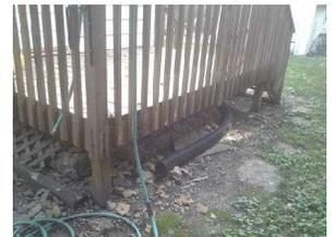
3. Grading: Minor slope, Negative slope - Grading has settled in areas around the home, allows moisture to accumulate near structure. Recommend repair by a qualified landscape contractor.
