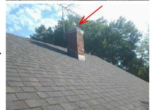
9. East, Center Chimney Flue/Flue Cap: Mortar - :Chimney flue cap is not installed. Recommend installation of rain/snow cap to keep moisture and wildlife from entering chimney flue.
