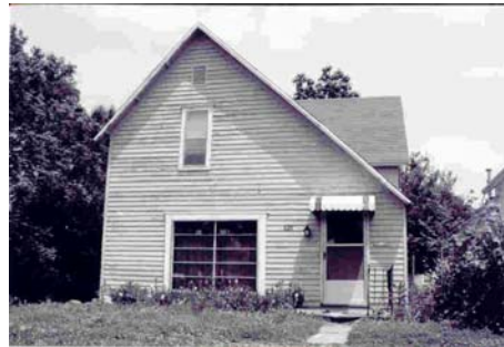
Inappropriate Porch and Window Alterations, 826 Rhode Island Street (Photo # 81)
