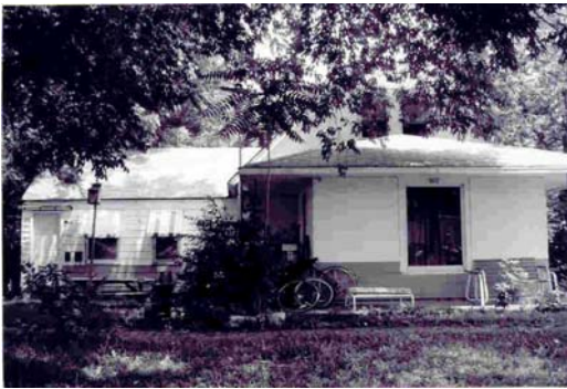
Inappropriate Addition and Windows, 822 Rhode Island Street (Photo # 80)
