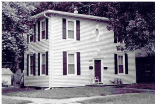
Vinyl Siding and Inappropriate Window Replacement, 1000 Rhode Island Street (Photo # 6)
