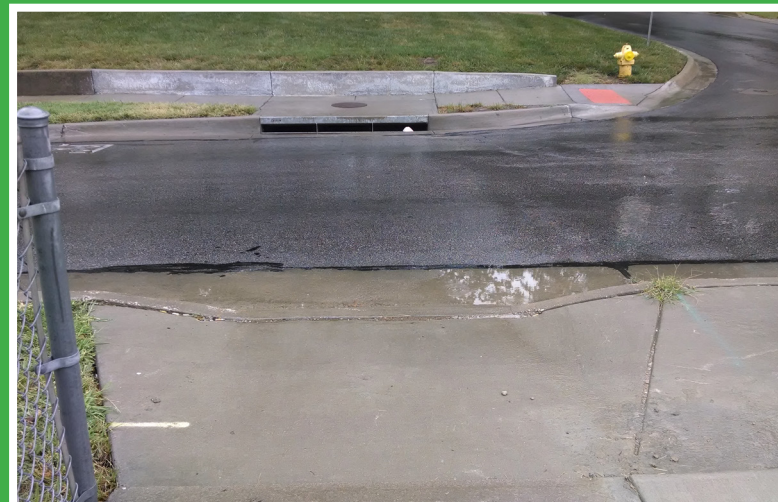
Figure 5-16: (Below) Naismith Drive – Curb Ramp Accessibility Issues.
