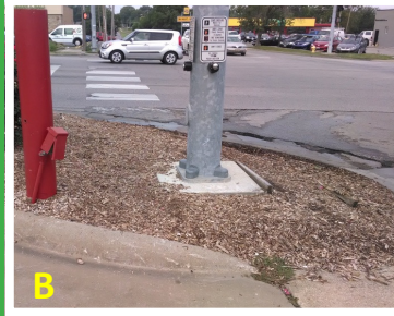
Fig. 6-7: Iowa & 9th Streets; SE Corner Featuring No Curb Ramps or Pedestrian Route
