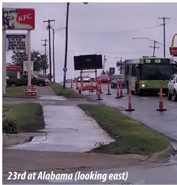
Figure 5-4: Examples of Key Sidewalk Segments along 23rd Street
