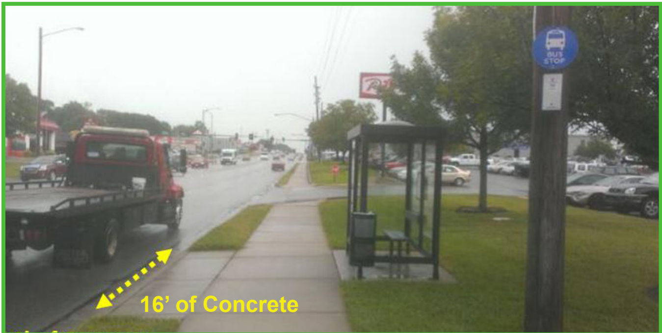
Figure 5-7: Example of Wide Concrete Boarding Area
