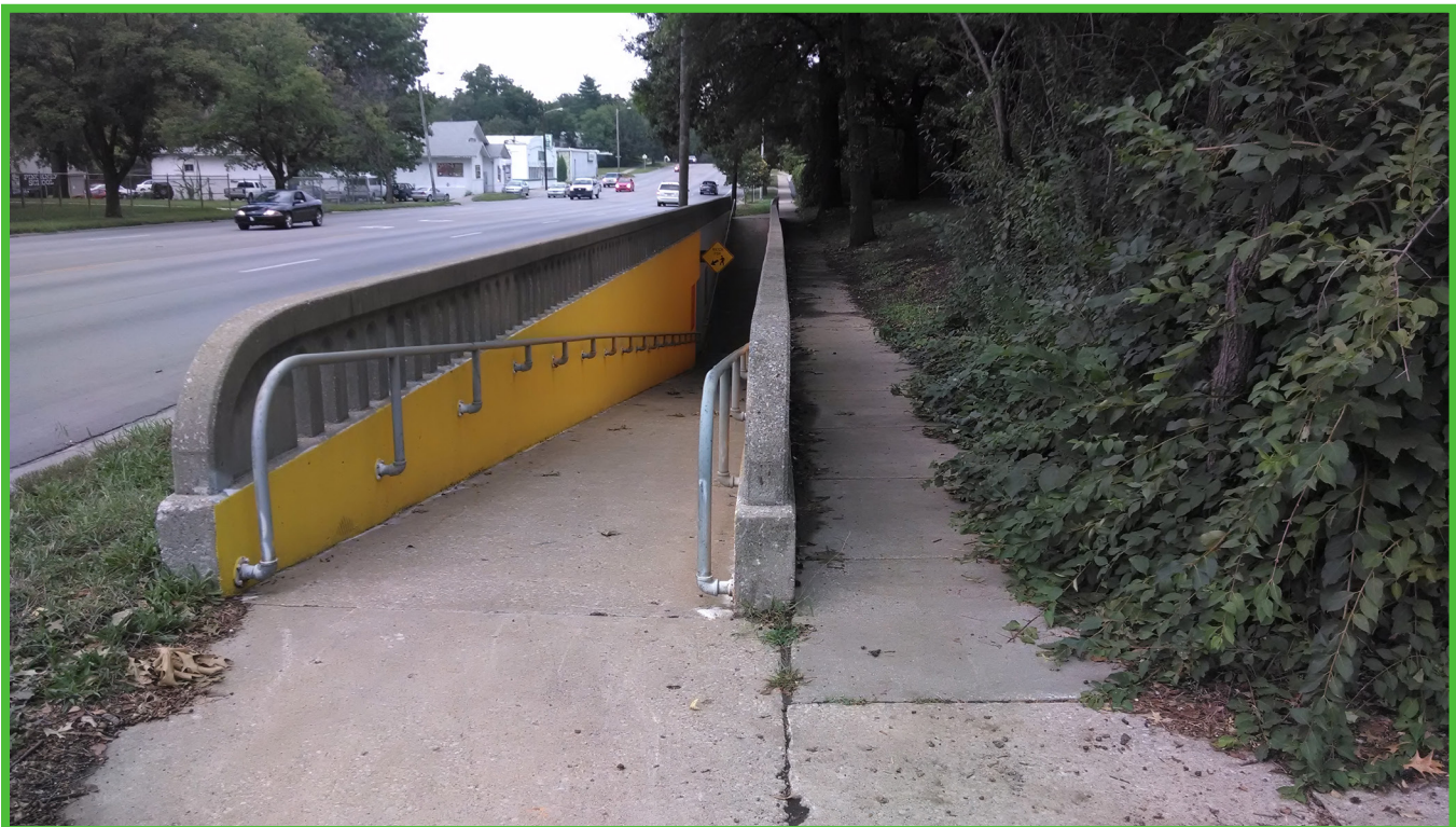
Ramp leading to the 6th Street underpass
