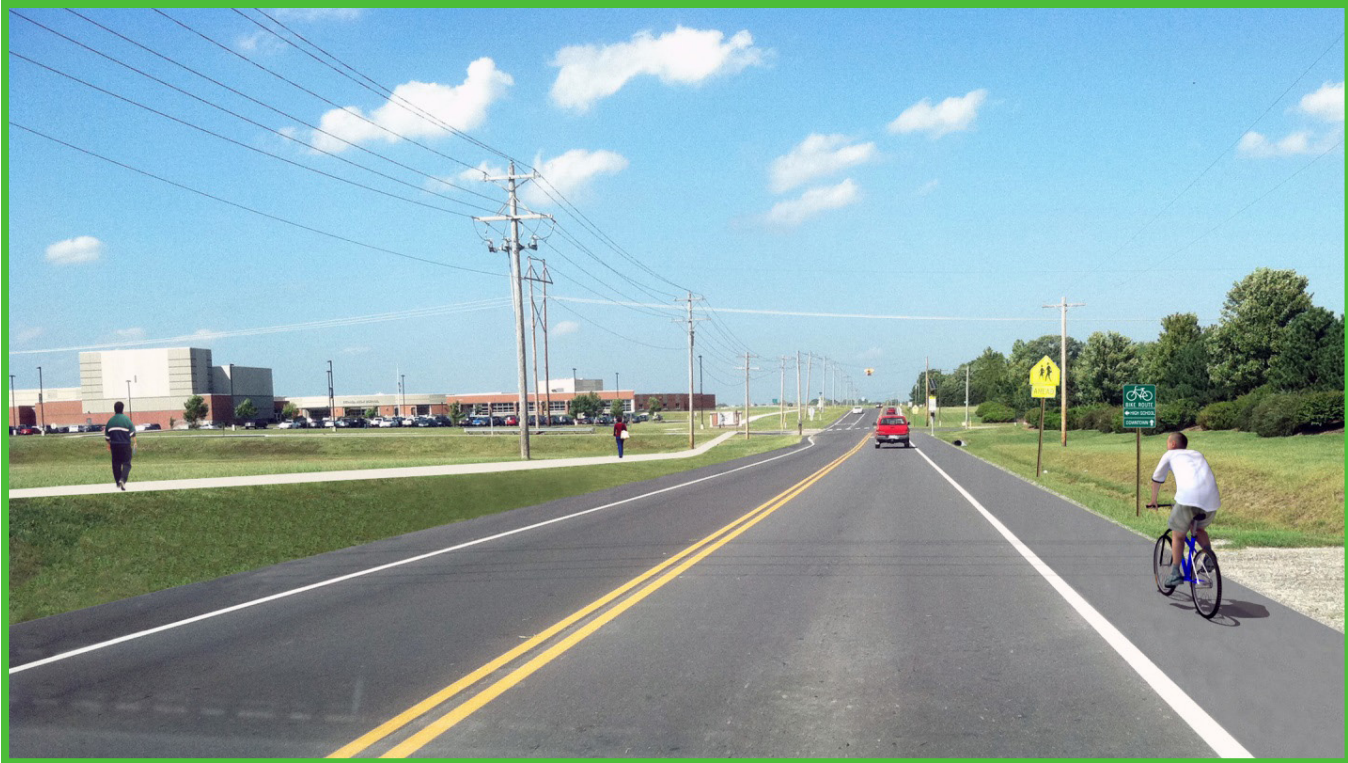
Photo rendering of paved shoulders and path added to County Route 1061 / Church Street in Eudora
