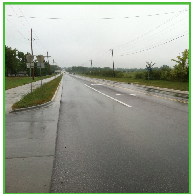
New path in Baldwin City along 6th Street
