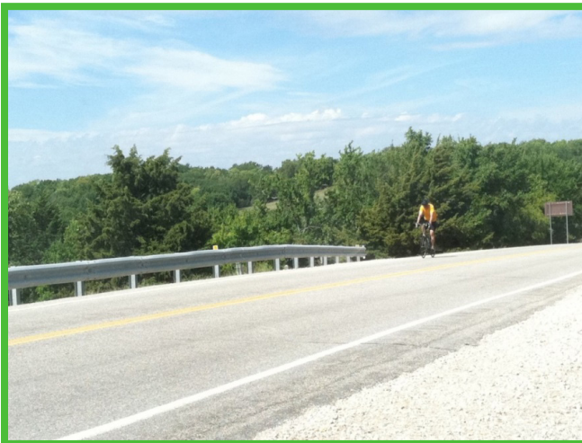
Bicyclist traveling south on E 900th Road across the impoundment
