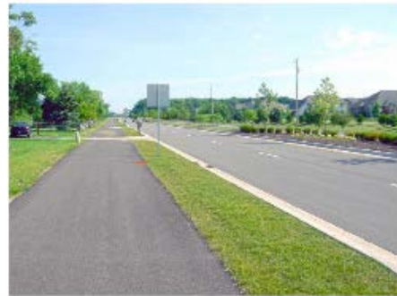
Figure 7: Example of Side Path
