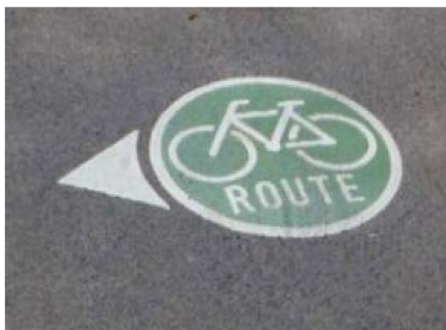
Figure 20: Example of 18-inch diameter thermoplastic marking on asphalt
