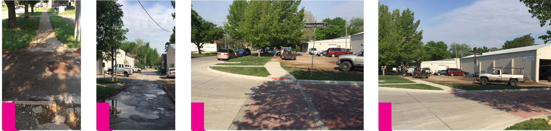
New Jersey to Pennsylvania north side of street
