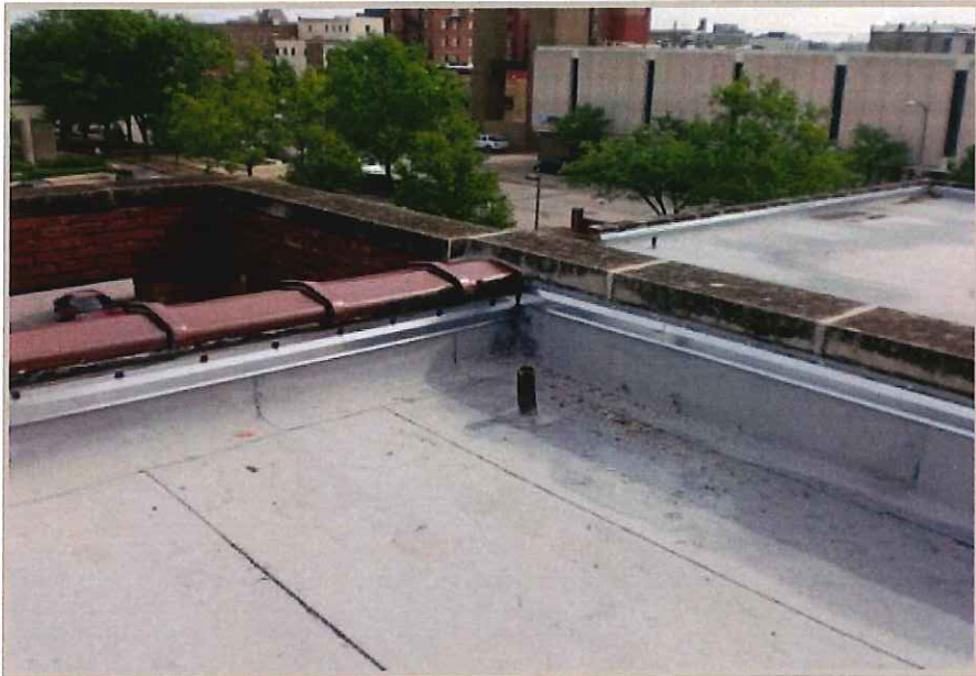
This section drains well and is in good shape.
