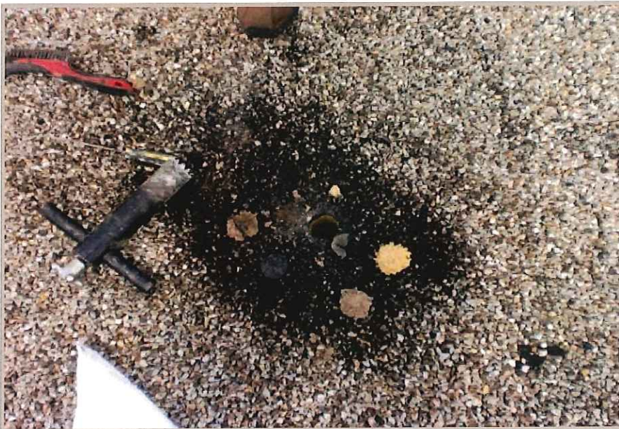
Core cut identifying the roofing elements.
