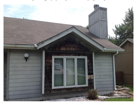
South elevation, rotten chimney chase
