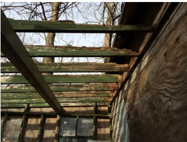
Interior (rear porch)
