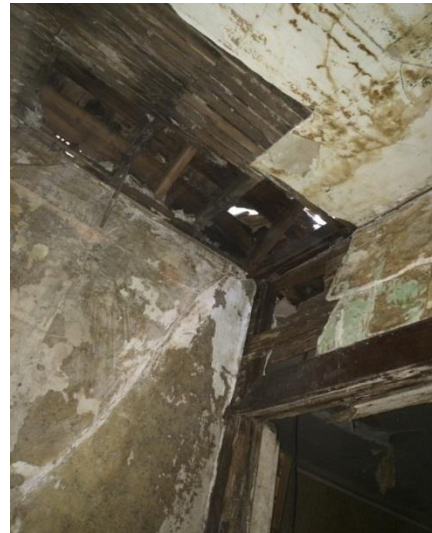
Front/south room – Ceiling rafters
