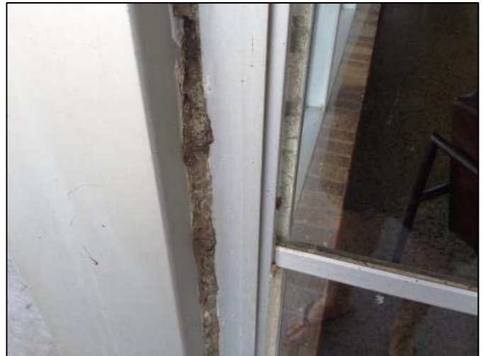
Caulk at exterior window
