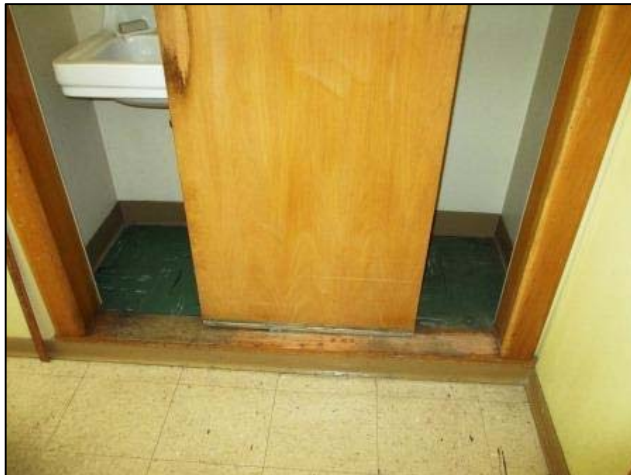
Agents office floor & closet 9x9 floor tiles/mastic under all tiles
