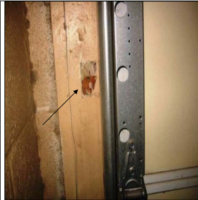
Deteriorated LBP on the baggage room A wall garage door casing.
