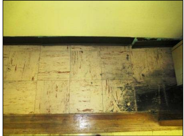
Freight office closet 9x9 floor tiles/mastic
