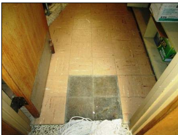
File room 9x9 floor tiles/mastic
