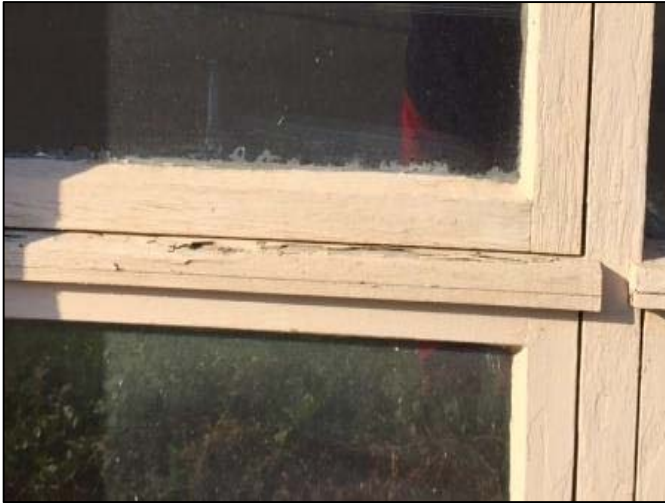
Window glazing on wood windows at exterior of freight office
