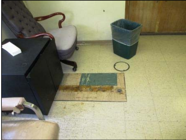
Freight office floor 9x9 floor tiles/mastic under all tiles
