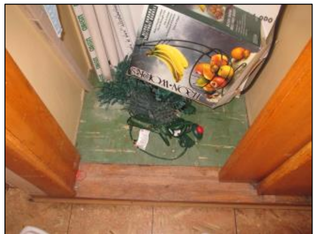
Ticket office closet 9x9 floor tiles/mastic
