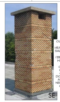
CUT OUT AND REPLACE ALL STRETCHER COURSES; HEADER COURSES TO REMAIN. SALVAGE BRICKS FOR REUSE AT REPAIR LOCATIONS (BELOW ROOF) AT EXTERIOR WALLS AS INDICATED. LAY NEW BRICKS TO MATCH COURSING AND EXISTING UNITS BETWEEN HEADER COURSES. CHIMNEY IS A DOUBLE WYTHE BRICK WALL AND REMAINING MASONRY NEEDS TO BE BRACED UNTIL CHIMNEY WALL IS FULLY RESTORED
