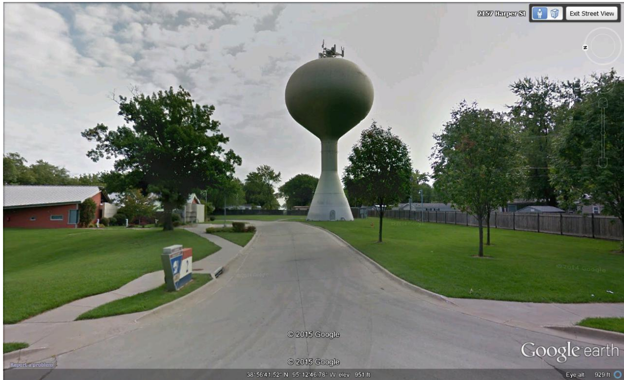
Harper Water Tower
