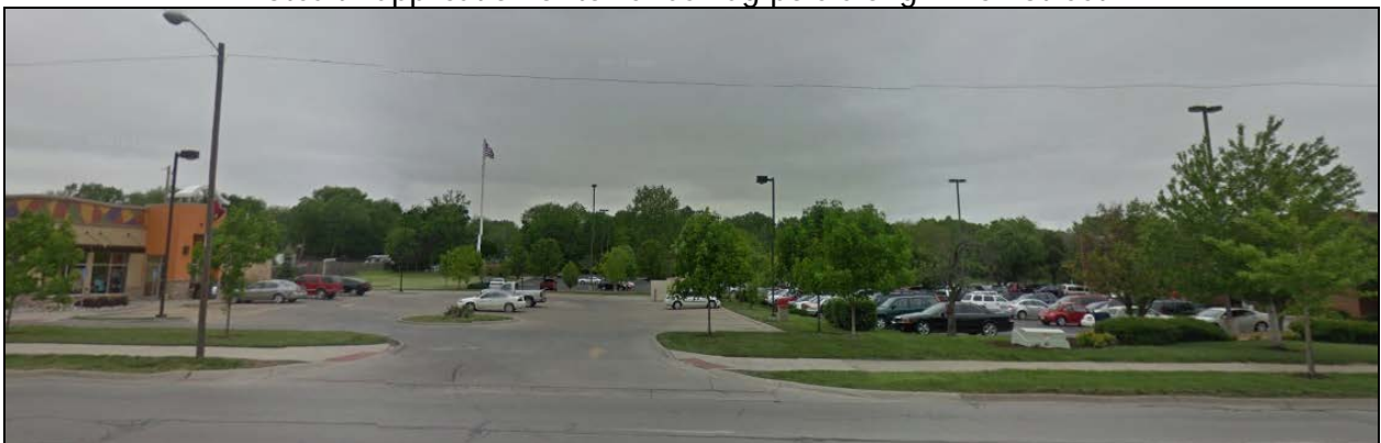
Figure 8: Existing Tower on W. 6th Street
