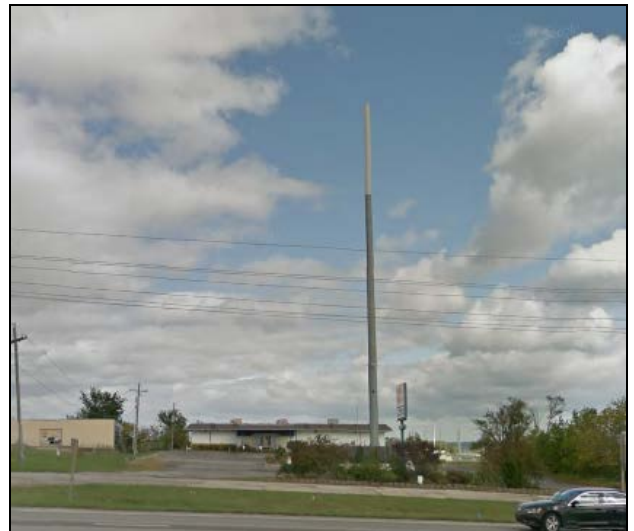
Figure 7: Existing Tower E. 23rd Street
