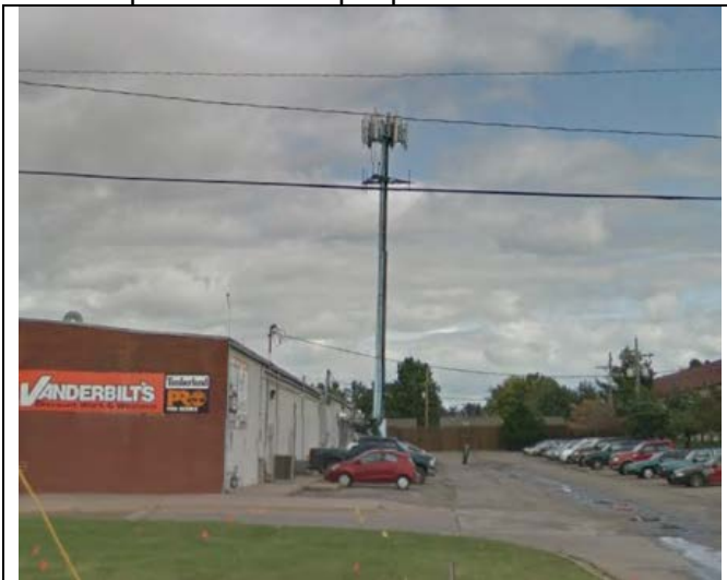
Figure 6: Existing Tower E. 23rd Street
