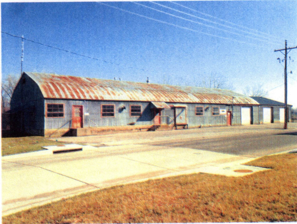
View of 620 E. 8 th Street, camera facing northeast
