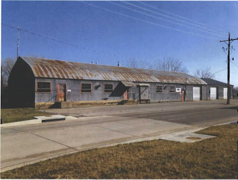
View of 620 E. 8 th Street, camera facing northeast
