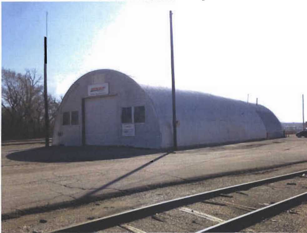
View of Quonset Hut 02, camera facing southeast
