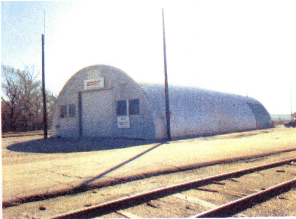
View of Quonset Hut 02, camera facing southeast
