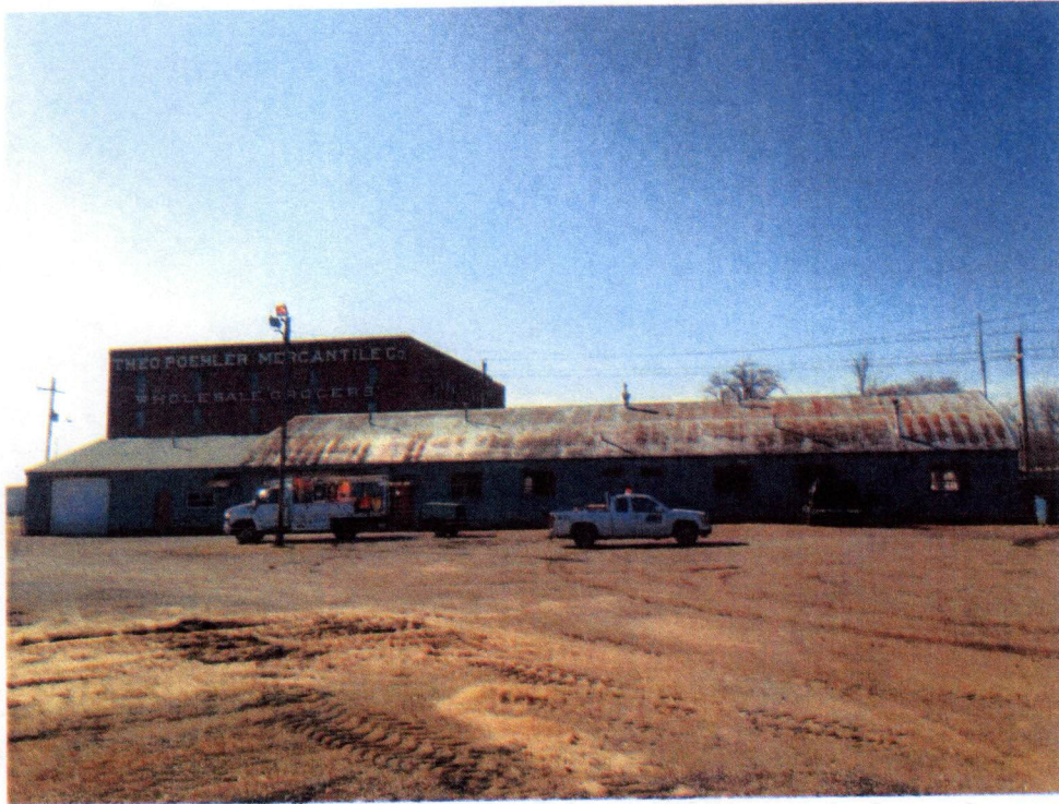
View of 620 E. 8 th Street with NRHP-listed Poehler Mercantile Company in background, camera facing south
