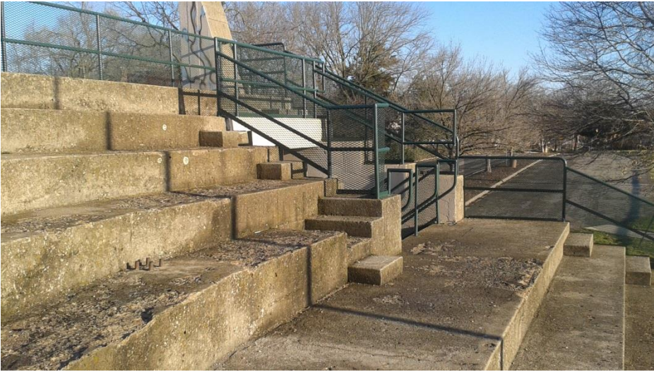
Hobbs Stadium – Repairs to concrete steps $20,000
