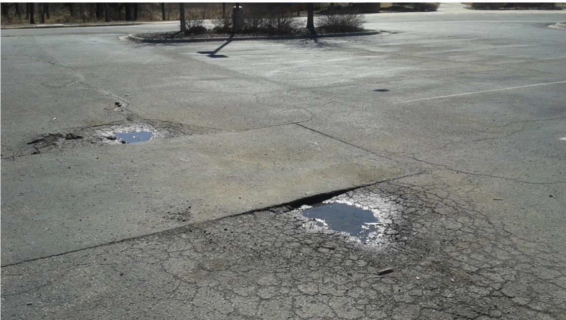
Clinton Lake Softball Complex Parking Lot Patch, Seal, Stripe $30,000
