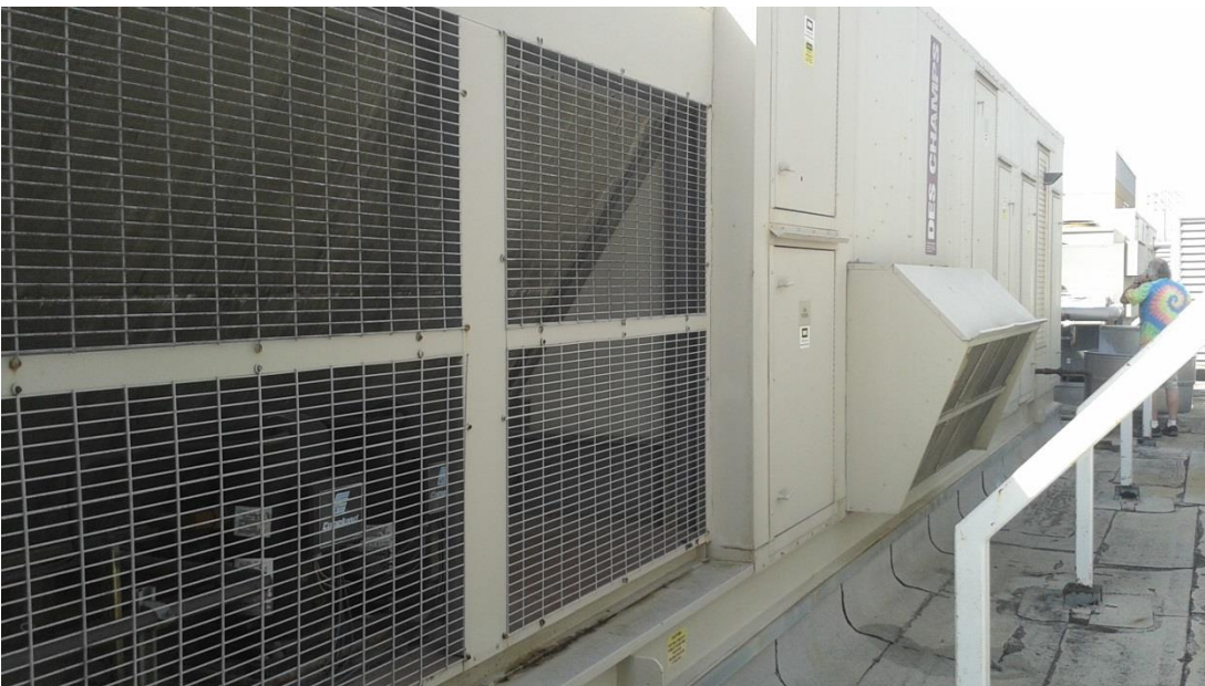
Indoor Aquatic Center – Replace HVAC unit for Leisure Pool $250,000
