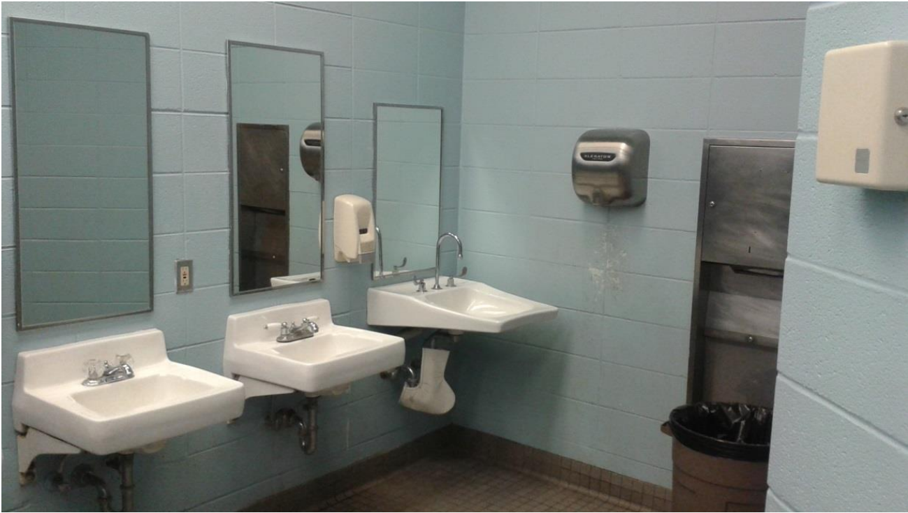
Holcom Park Center – remodel women's restroom $25,000
