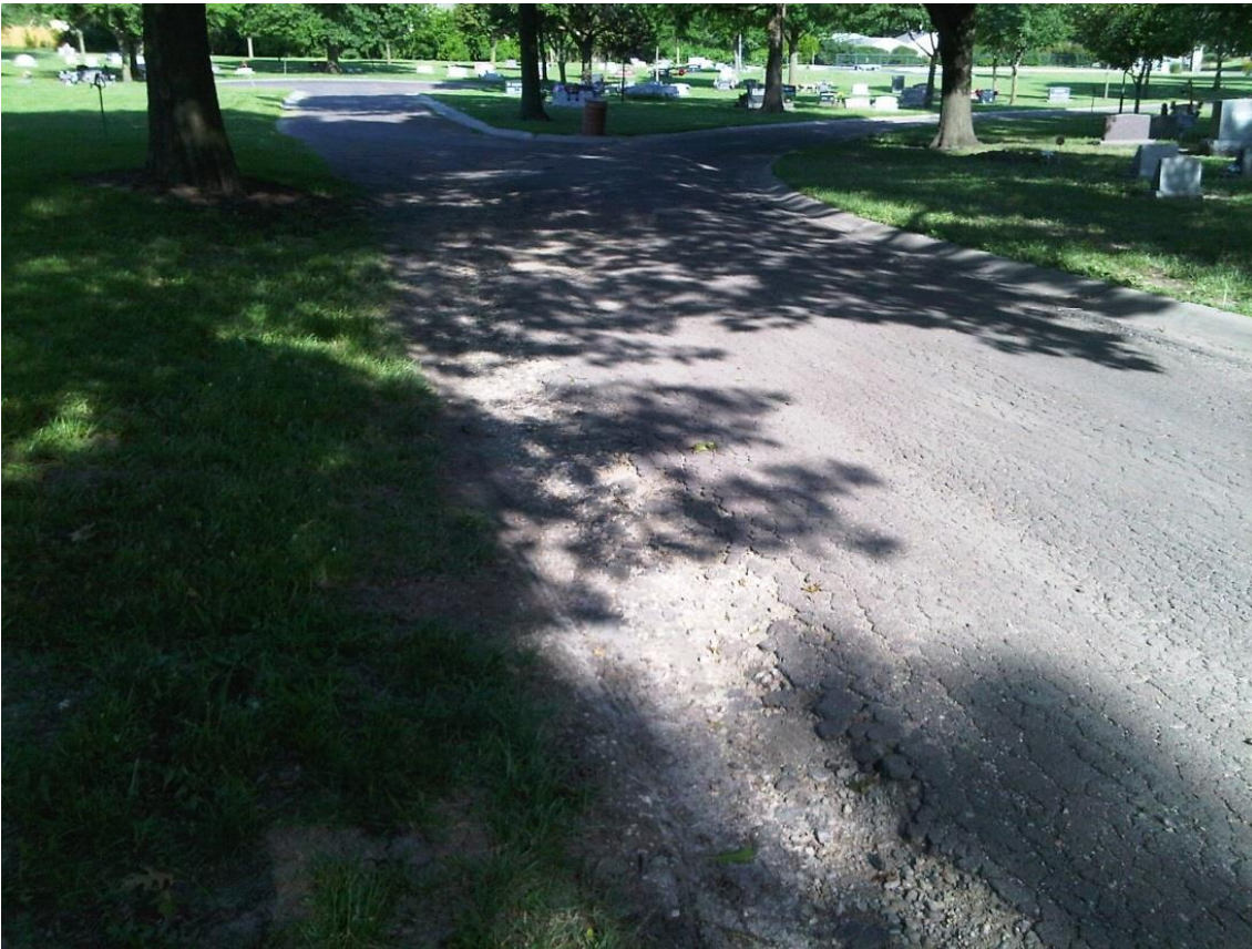
Oak Hill, Memorial Park, Maple Grove Cemeteries - Road repair - $60,000
