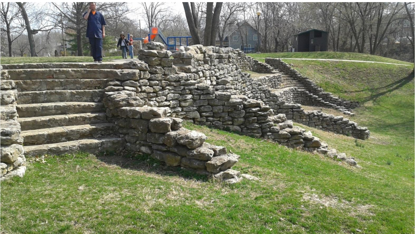
Clinton Park – Clean and tuck-point historic stone wall $40,000
