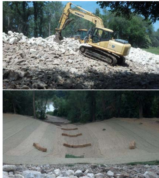
Work on Kansas River Levee
