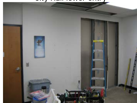
Door removed at Health Building
