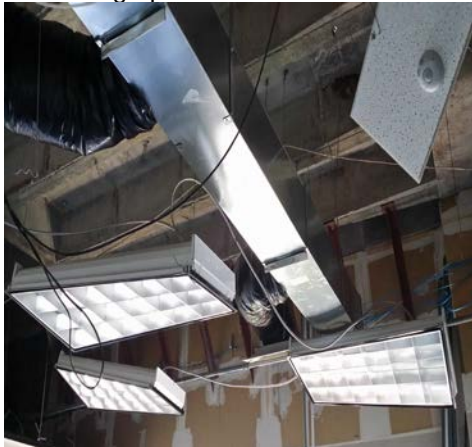
City Hall 4 th floor remodel
