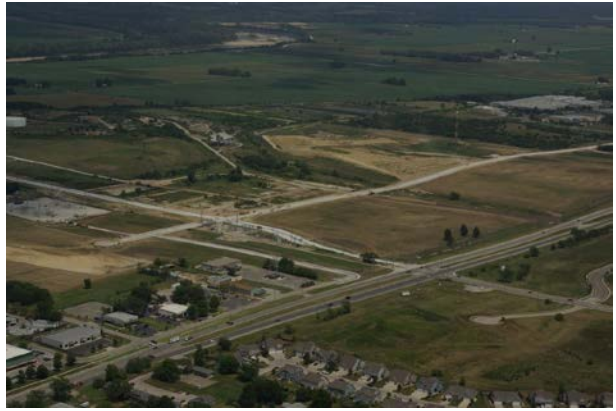
Venture Park infrastructure
