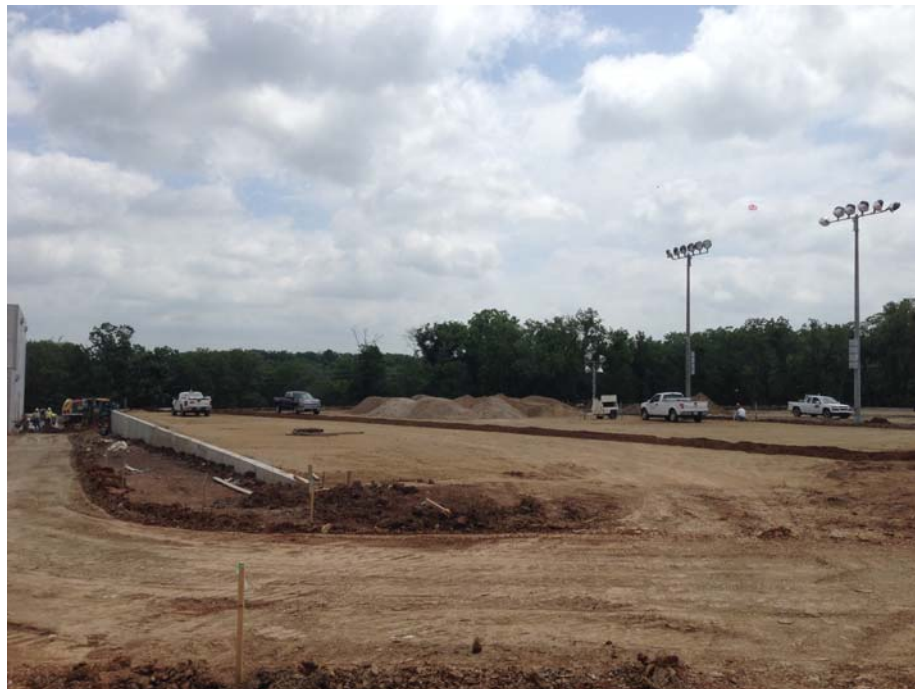
Beginning of tennis court construction
