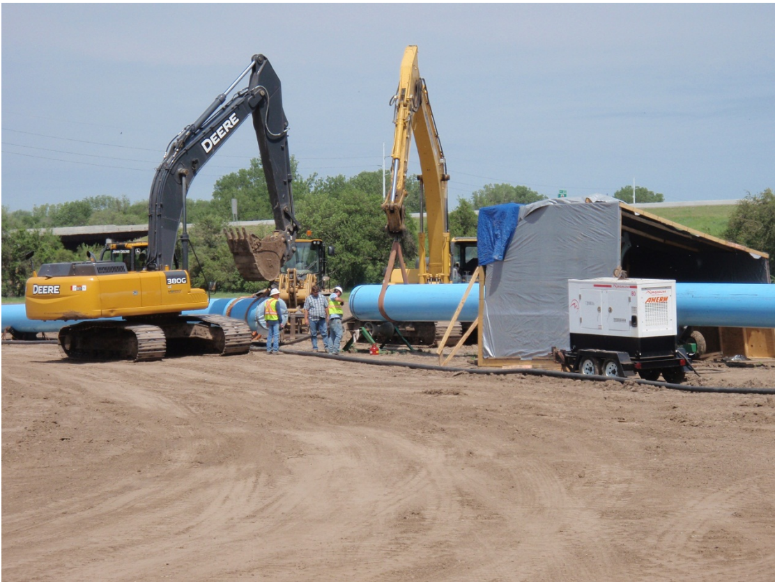
Pipe being positioned for fusing during the pull back.
