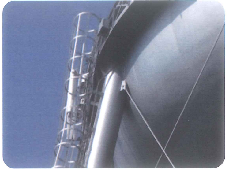
Exterior Ladder & Ladder Cage
