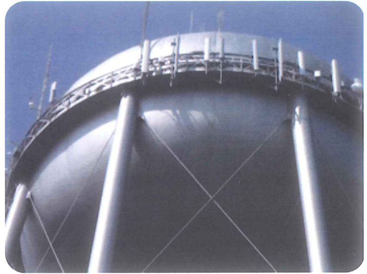
Catwalk Area, Top of Tank, & Antennas
