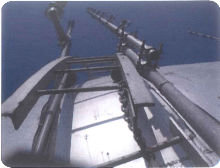
Rolling Ladder to Roof Top
