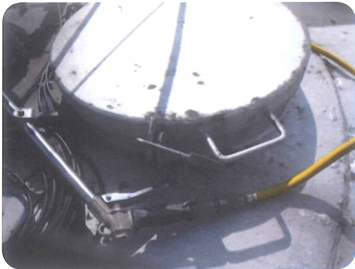
Upper Roof Hatch
