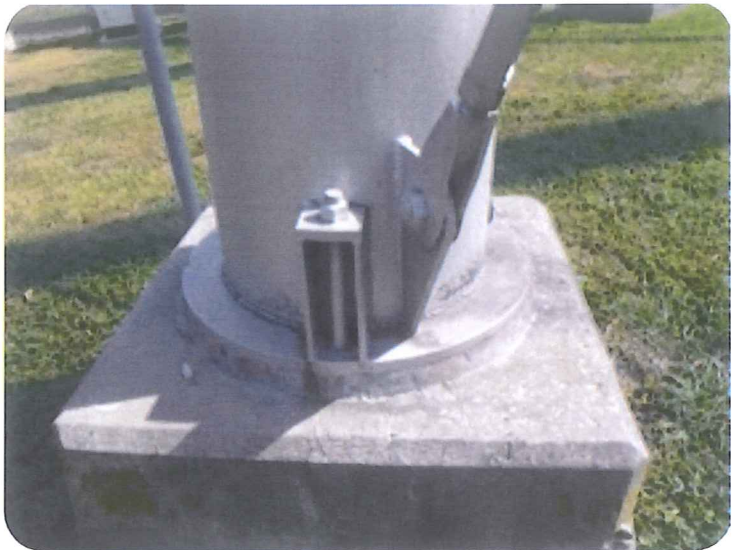
Anchor Bolts & Foundation
