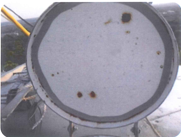
Roof Hatch Gasket
