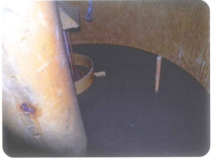
Overflow Pipe/Sludge in bottom of Tank Prior to Cleaning
