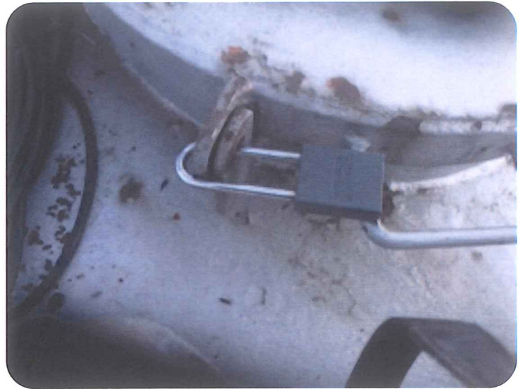
Upper Roof Hatch with Lock
