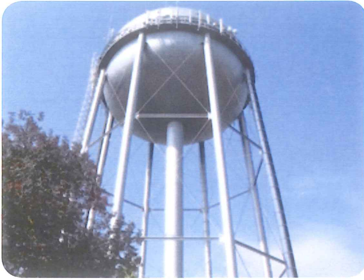
Lawrence, KS, 500,000 Gallon Elevated Water Tower
