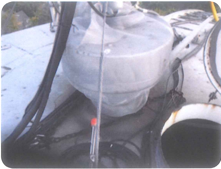
Vent System with Temporary Screen Wrap
