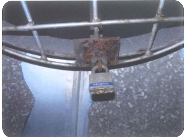
Ladder Cage Locked
