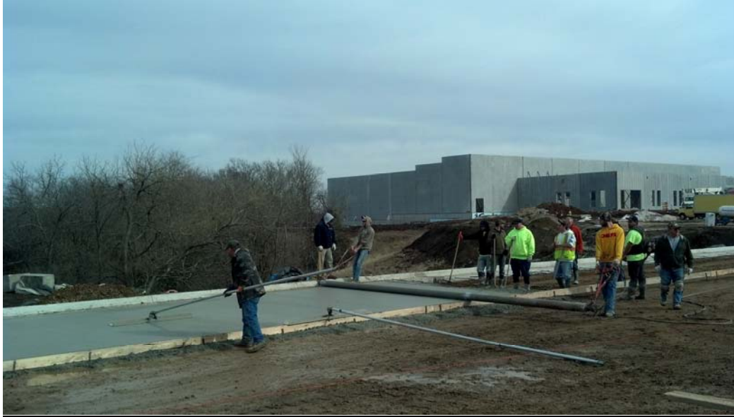
Interior parking/bus lane concrete pour in February
