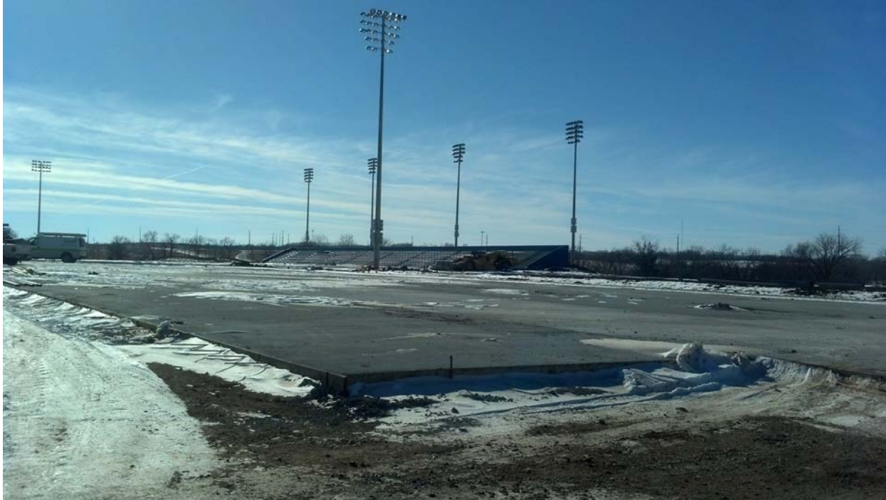
Parking lot north of Track Facility
