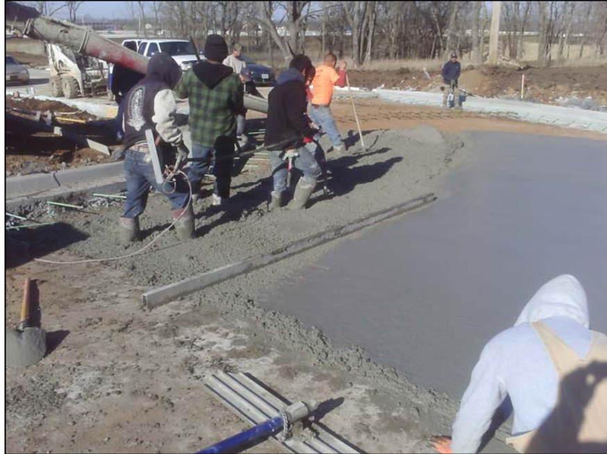
Vibrating concrete.
