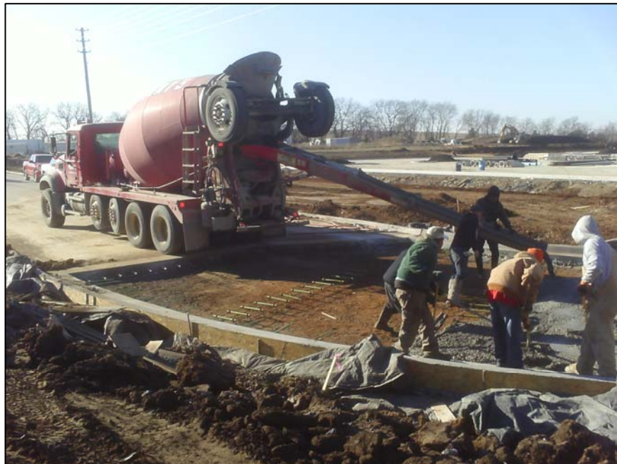
Began placing 10" concrete pavement.
