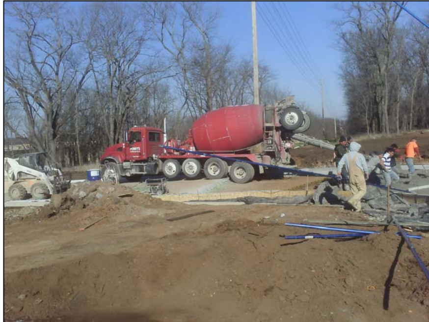
Backing ready-mix truck over smooth dowels.
