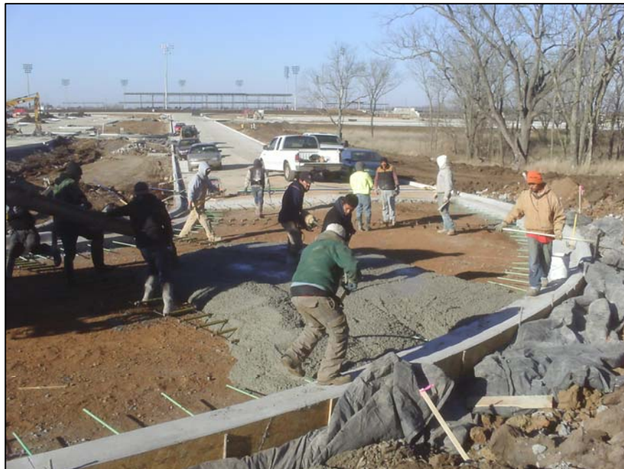
Placing concrete.
