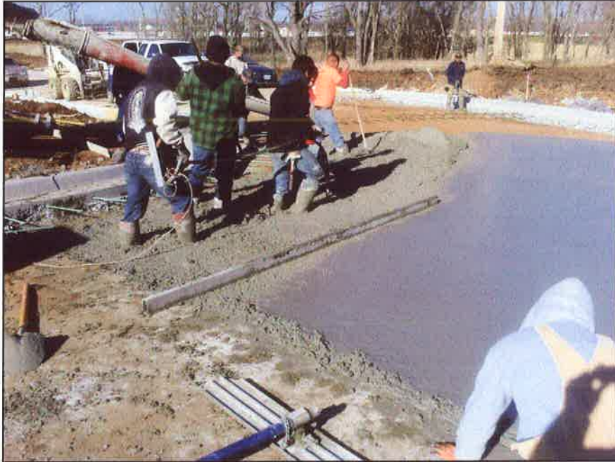
Vibrating concrete.
