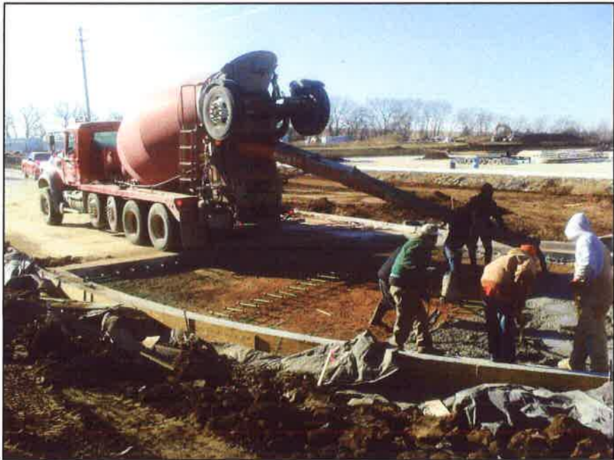
Began placing 10" concrete pavement.
