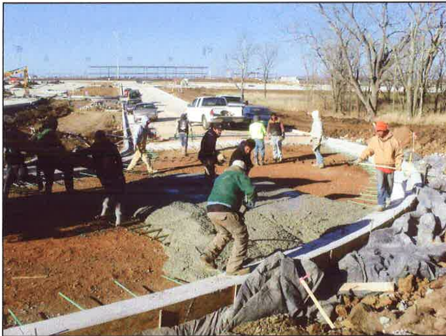
Placing concrete.
