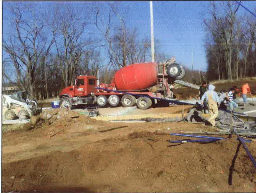
Backing ready-mix truck over smooth dowels.
