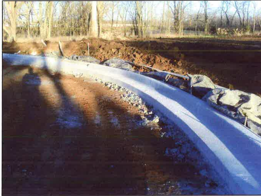
No tie bars. Requested Contractor install epoxy coated bar to be drilled and grouted.
