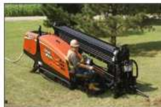
Horizontal Drilling Eliminates Trenches
