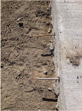
Longitudinal tie-bars on GWW
