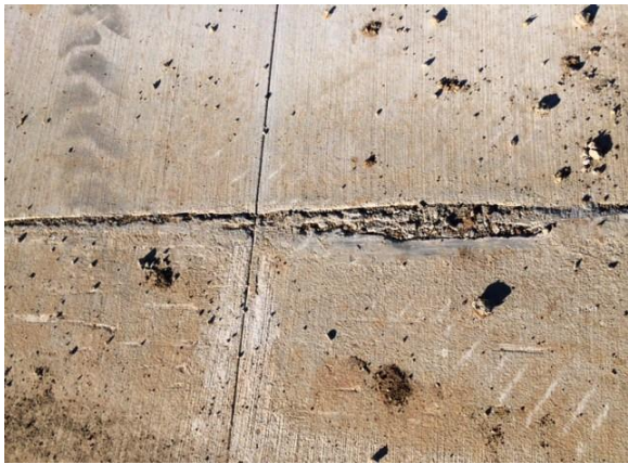
Joint Spalling
