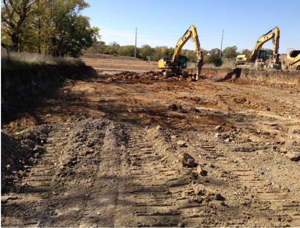
Grading & rock excavation for Rock Chalk Drive
