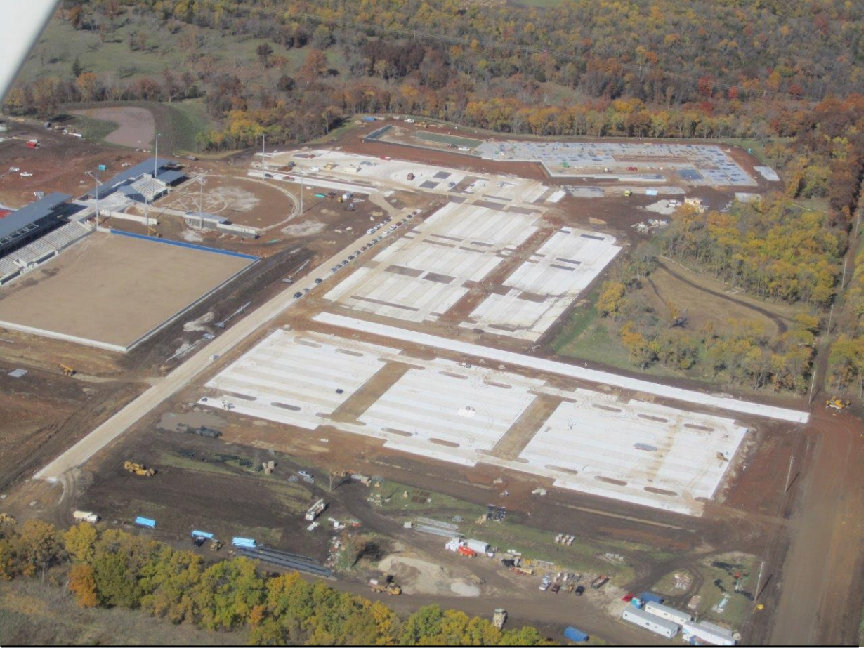
Work complete through October
