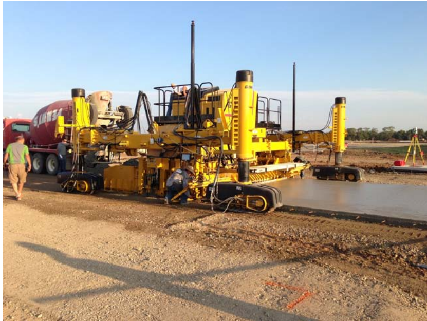
Concrete parking lot paving
