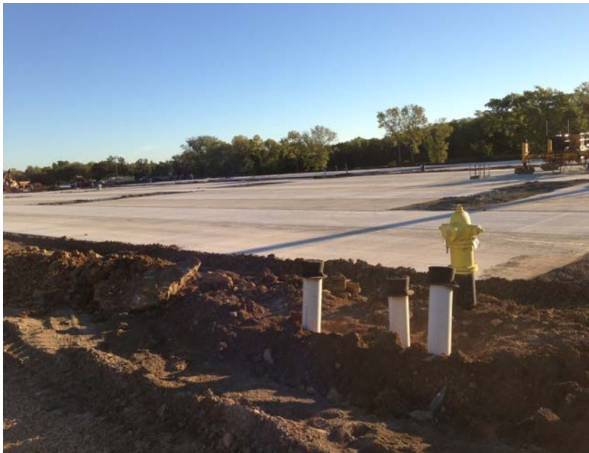
Concrete parking lot
