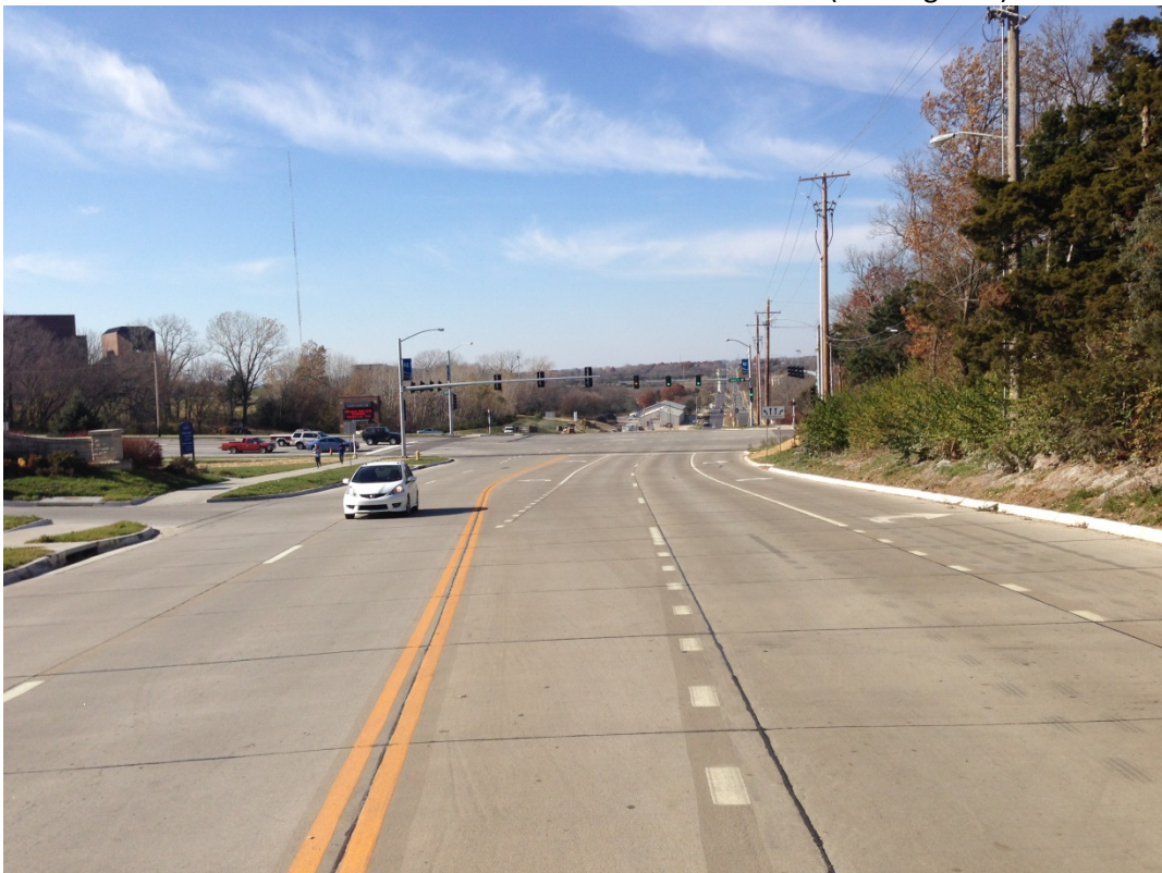
BBP Additional Turn Lanes (looking West)
