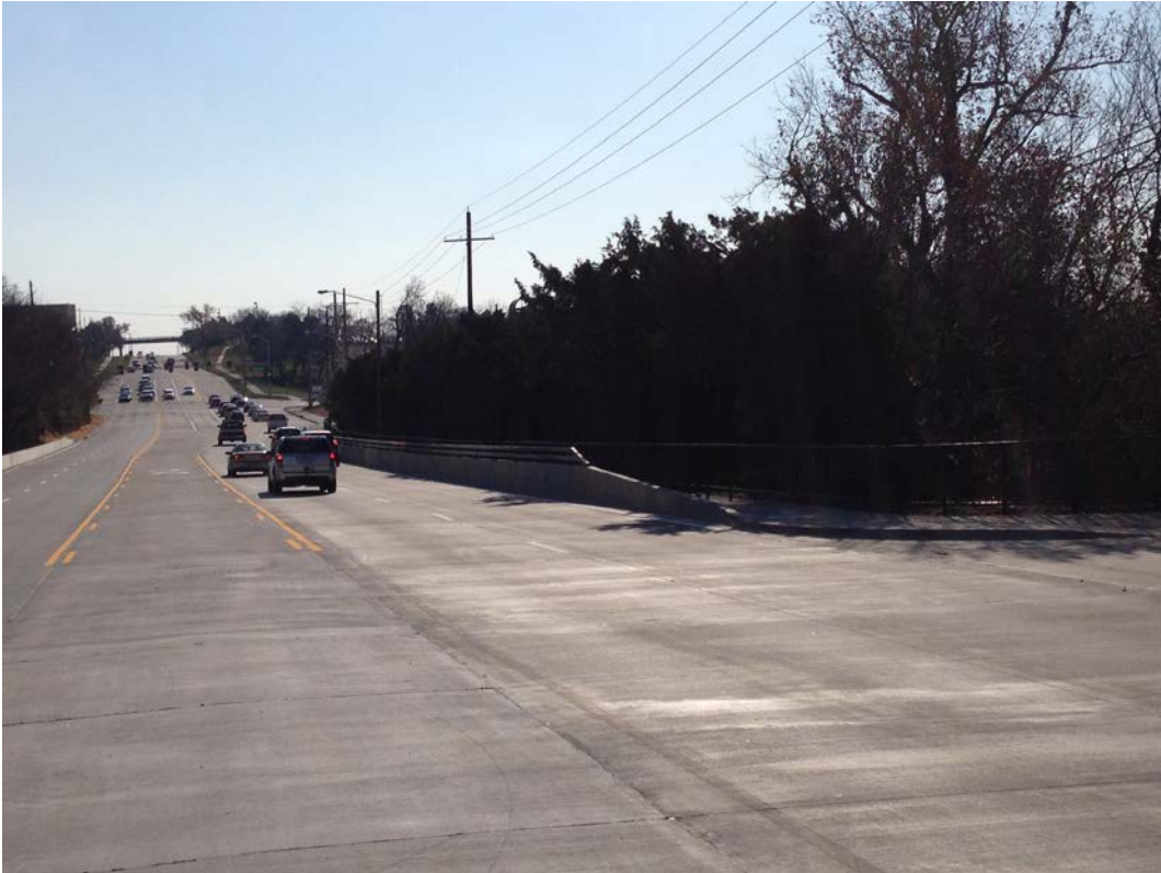
Iowa Barrier Protection Wall and Hand Rail (Looking South)
