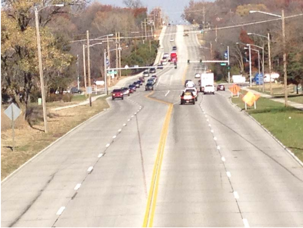
Iowa – Additional Left Turn Lanes (Looking North)
