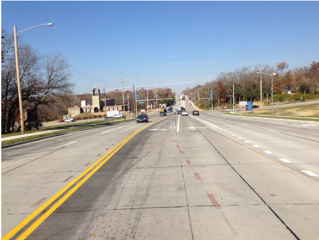
Iowa Additional Turn Lanes (Looking North)
