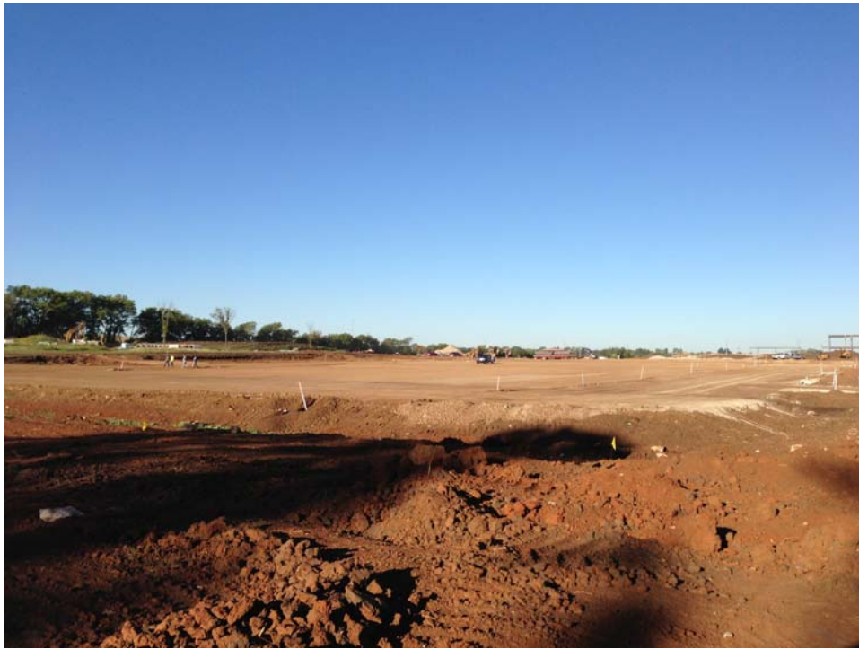
South parking lot finish grade with subgrade treatment
