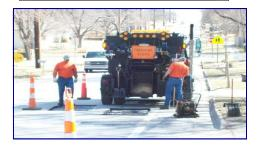
**What Is A Pothole?** While several factors contribute to the creation of potholes, they are distresses in the pavement that can create a failure of the pavement. This failure causes the pavement material to crumble and create a void in the pavement.
