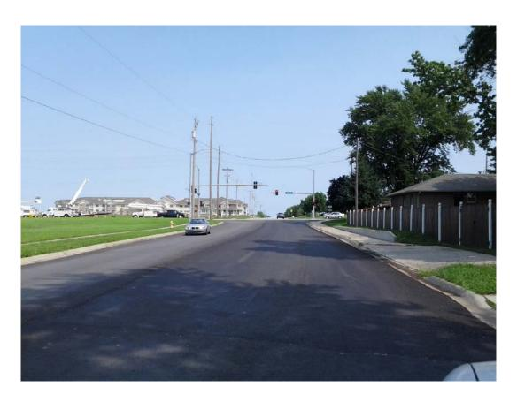
Folks Rd (south of 6<sup>th</sup> St) – after patching/ reapplication of surface seal by machine
