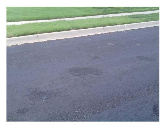
Lili Dr - example of power steering marks with loss of seal, completed with minor patching
