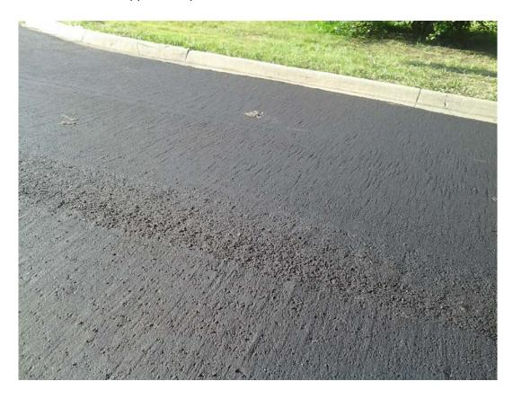
Example of microsurface seal with rougher texture than a roller compacted 2" mill and overlay; Over time and with traffic, the material will tend to smooth out more
