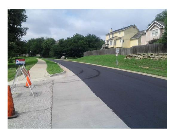
Inverness Dr – example of seal damage from aggressive vehicle turn near a temporary road closure
