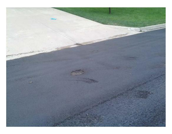
Vantuyl Dr – example of power steering marks, some leading to complete loss of seal requiring minor patch
