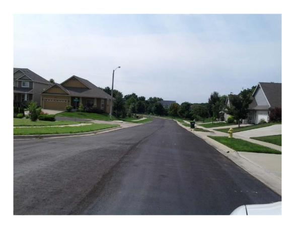
Larissa Dr near cul-de-sac – rougher texture apparent but typical in bulb areas where there is overlap of the application passes of the surface seal machine
