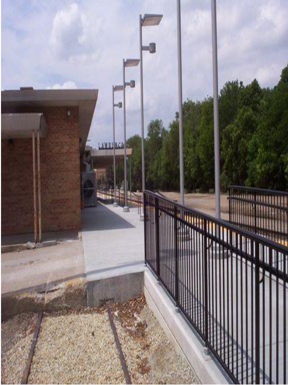
Exterior the platform improvements on north side of station 04MAY2012
