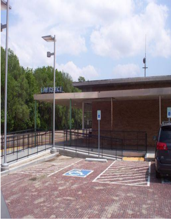
Exterior showing part of the platform project improvements 04MAY2012
