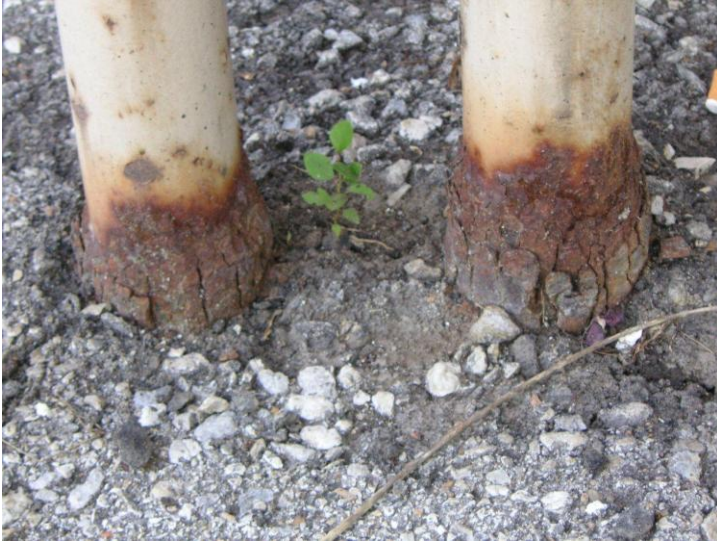
Canopy columns 16September2009
