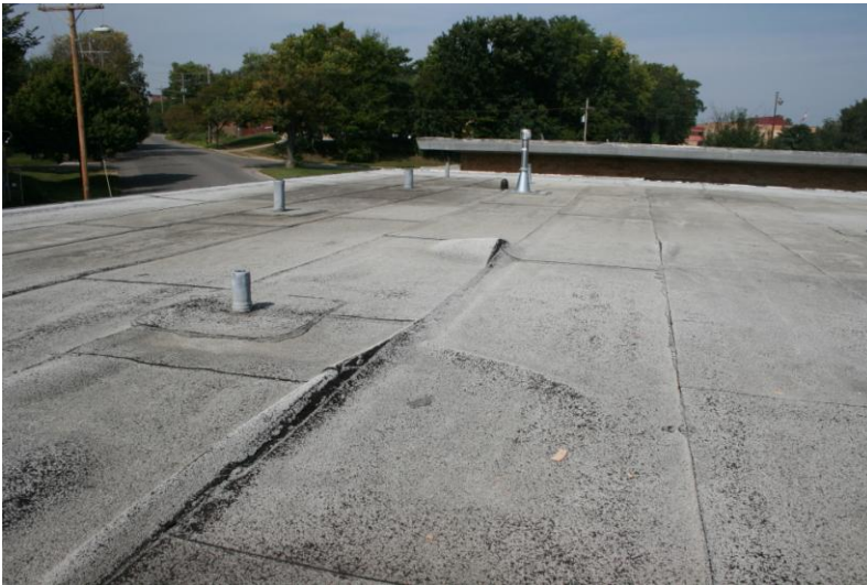
Roof looking west 16September2009
