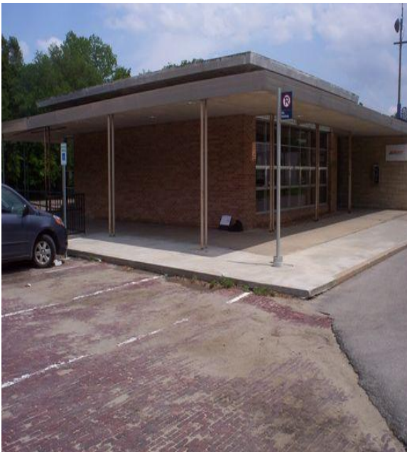
Exterior showing part of the platform project improvements 04MAY2012
