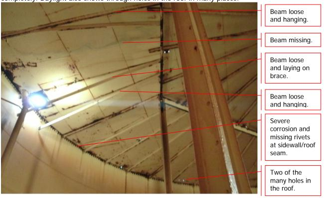
72 beams support the roof, 24 on the interior ring and 48 on the exterior ring. All have varying degrees of corrosion.
