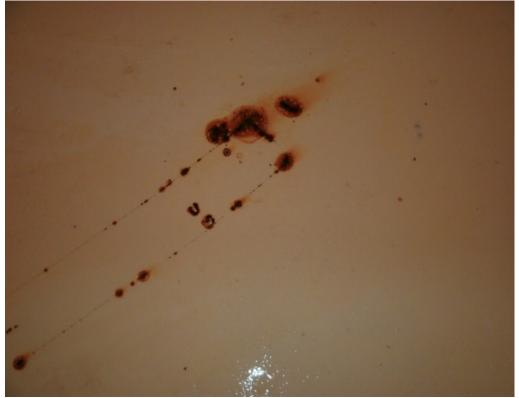
Corrosion near the sidewall/floor seam, potentially the cause of a leak in the tank.
