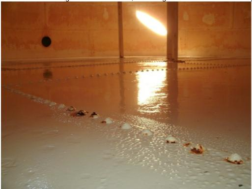
Corrosion caused by the missing roof beam that possibly fell and lay on the floor of the tank.
