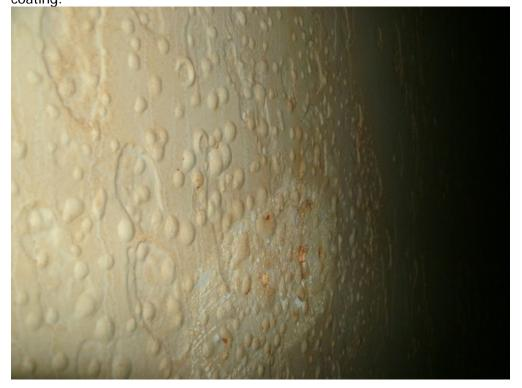
Severe corrosion and coating failure as seen on the below beam as it attaches to the roof and sidewall.
