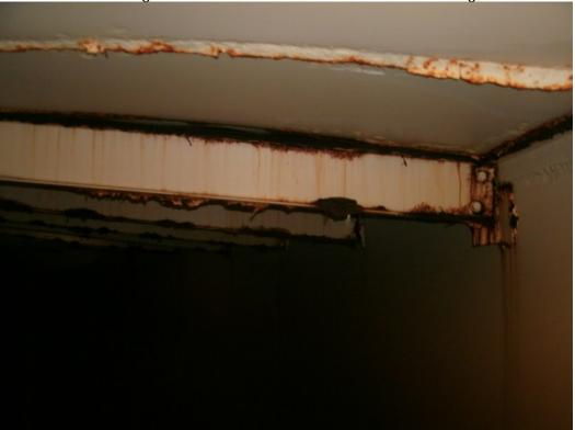
Coatings on the interior walls show severe blistering caused by moisture under the coating.
