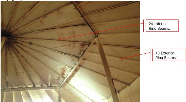
Corrosion of the rivets at the sidewall and roof seam has corroded into the metal.
