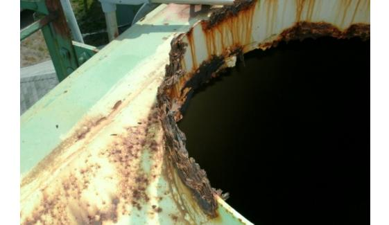
Roof beams show significant deterioration of the metal and coating, as well as corrosion.
