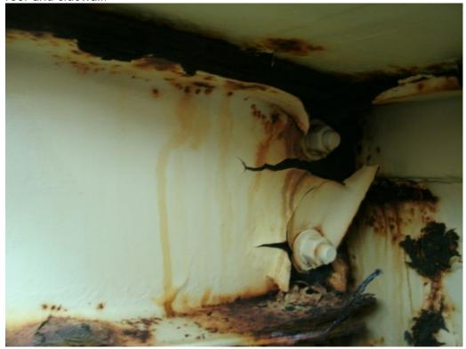
Corrosion has deteriorated coating causing metal loss of many of the roof beams.
