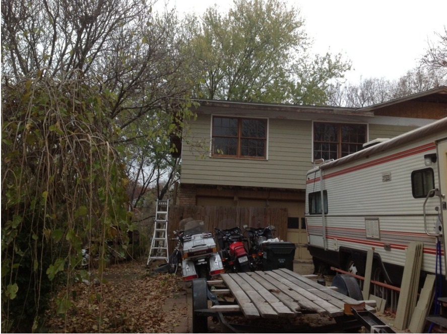
East Elevation (SE Corner)
