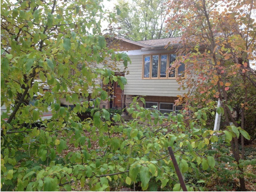
East Elevation (NE Corner)
