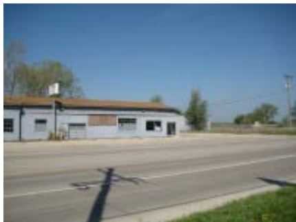
Former Kaw Metals, SW corner, TeePee Junction
