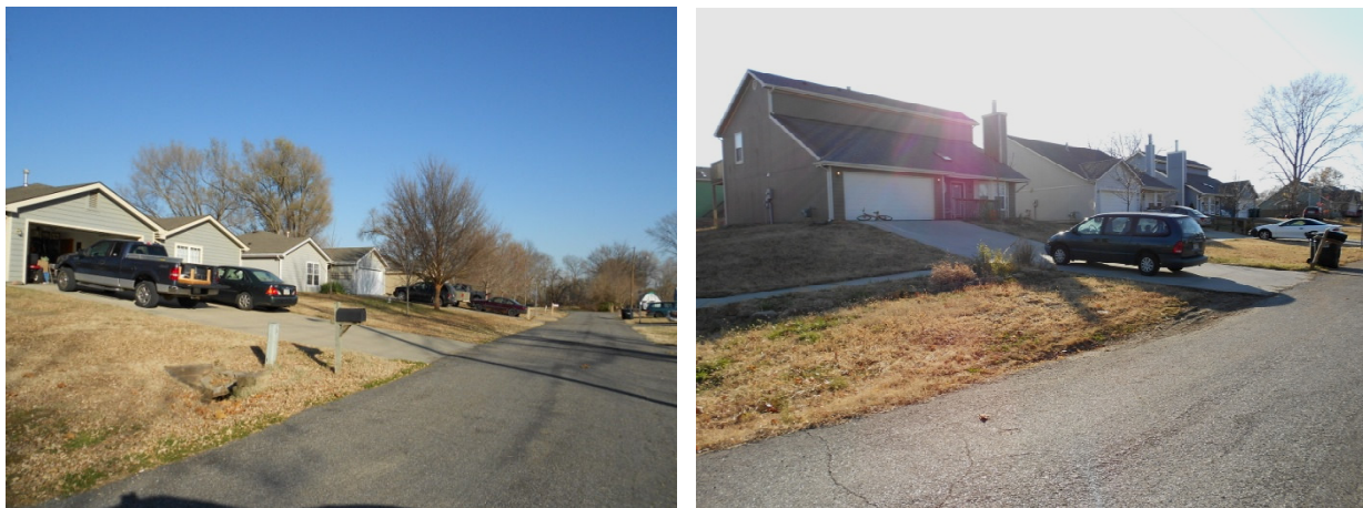
Figure 4 - New houses built on fill along the eastern half of the 700 block of Lake Street – an area that used to flood. Note the lack of culverts under drives in the photo on the right.
