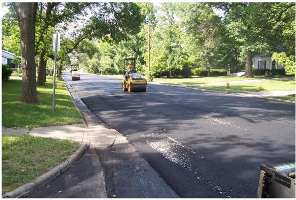
**Description** – Massachusetts St during applicatin of Asphalt Leveling Course as part of Contracted Asphalt Overlay.
