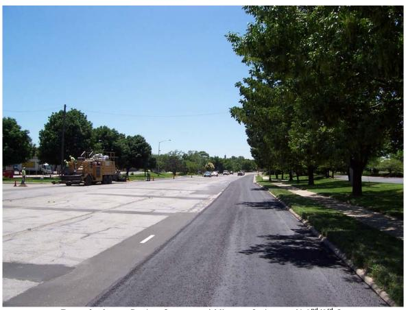
**Description** – During Contracted Microsurfacing on N 2<sup>nd</sup>/3<sup>rd</sup> St (Completed Asphalt Patching seen here also).
