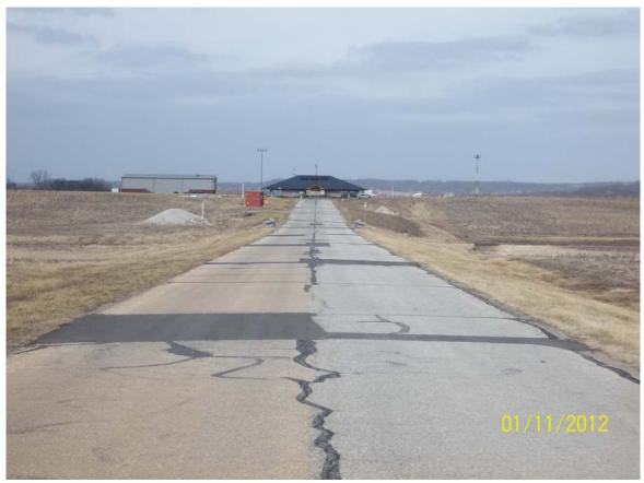
**Description** – Airport Rd prepared with Asphalt Patching prior to Contracted Microsurfacing.
