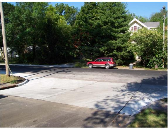
**Description** – Pawnee Ave at Massachusetts St after completion of Contracted Asphalt Overlay (Installed Concrete Intersection Approach seen here also).
