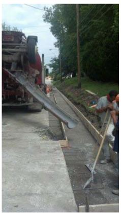
**Description** – During Contracted Concrete Patching & Curb Replacement on N 3<sup>rd</sup> St north of Maiden Ln.
