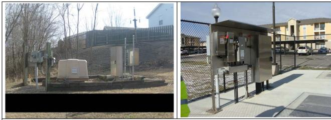
**Figure 3.** Existing pump station on the left. Example of new station (without the fencing) Underground facilities will be level-or slightly elevated and the panel will contain the above ground equipment.
