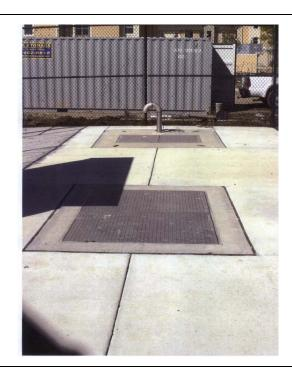
**Figure 3c.** Remainder of pump station is underground with exception of vent.
