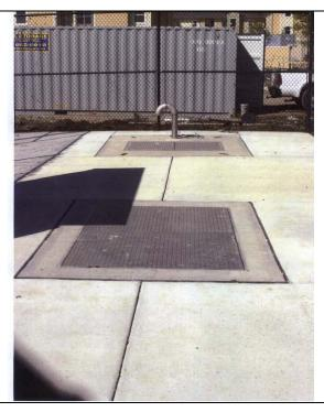
**Figure 2c.** Remainder of pump station is underground with exception of vent.
