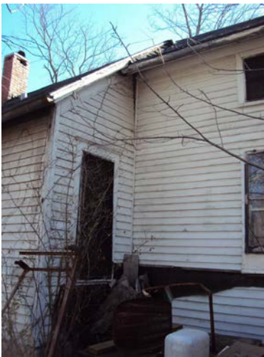
North wall, shows separation between original structure and addition
